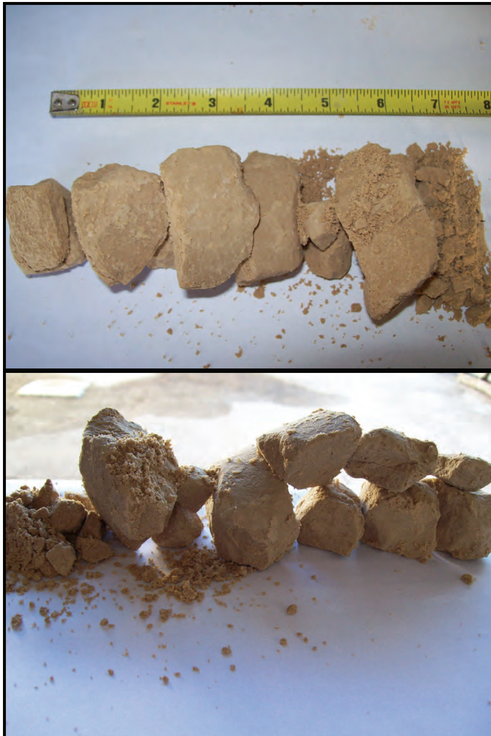
Photograph #1: Limestone Core RC-1, Boring B-19. Core Length Attempted: 6-in; Recovery: 4-in Consistency: Very dense (SPT N = 50/4" and 50/3" for the spoons above and below RC-1), but friable LIMESTONE
