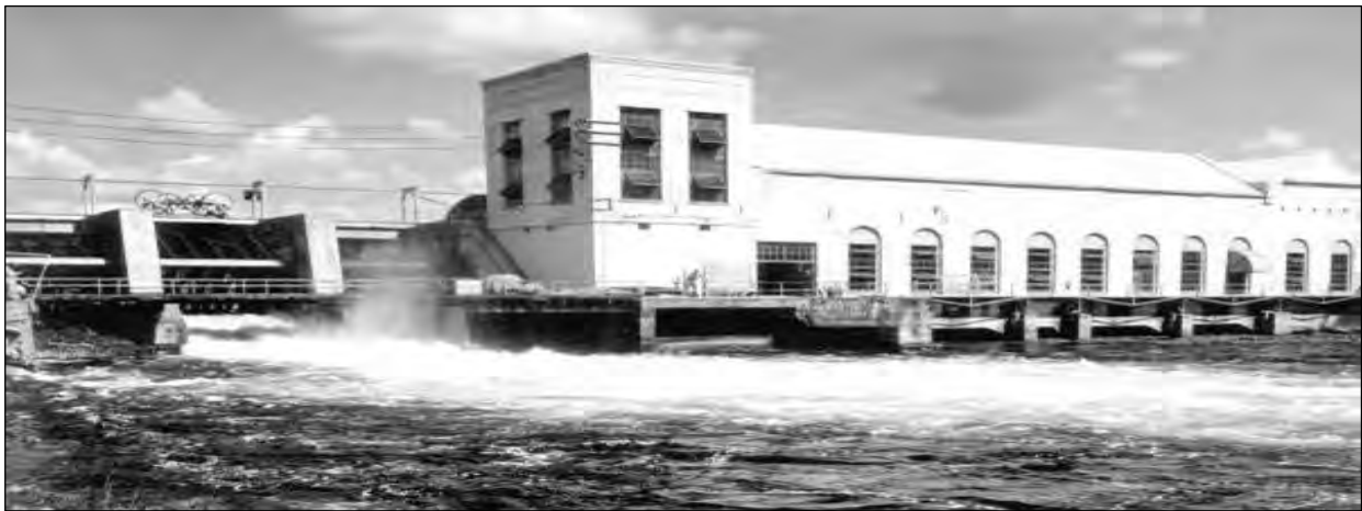
Figure 3.8. 1955 photograph of the Dunnellon Dam and Hydro-Electric Power Plant. Source: Florida Center for Instructional Technology, University of South Florida.
