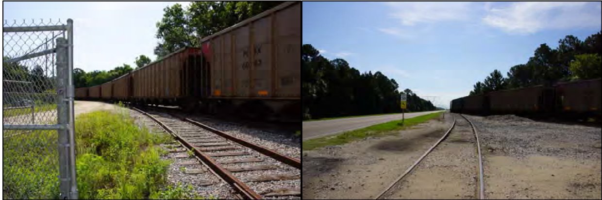
Figure 5.4. Views of resource 8CI01455. Left: View northeast along the loop at the western end of the spur line; right: View east along West Powerline Street on the south parcel boundary.
