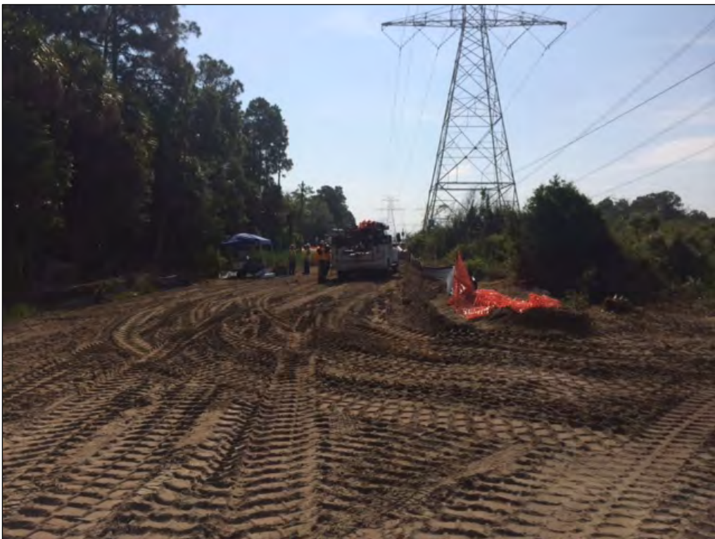
Figure 2.6. Activities within the transmission line on the DEF 2018 CC project area.
