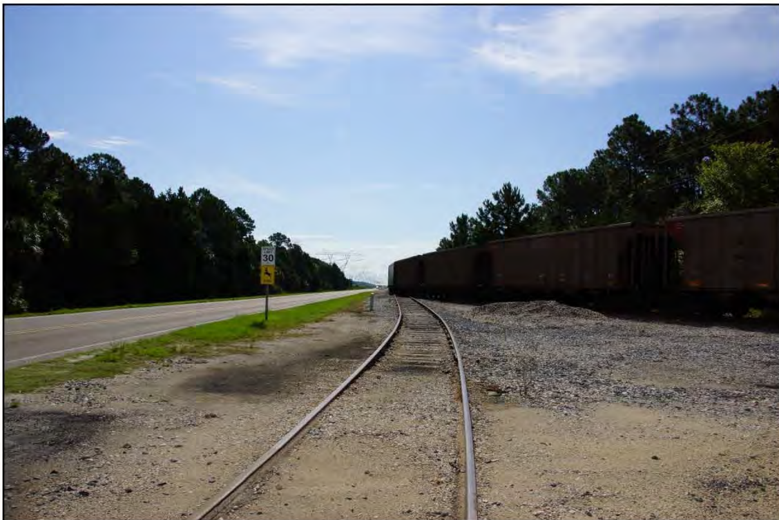
Views of newly recorded Linear Resource CI01455, Seaboard Coast Line Railroad, within the Duke Energy 2018 CC Survey Area in Citrus County, Florida. Top: View northeast along the loop at the western end of the spur line; bottom: View east along West Powerline Street on the south parcel boundary.
