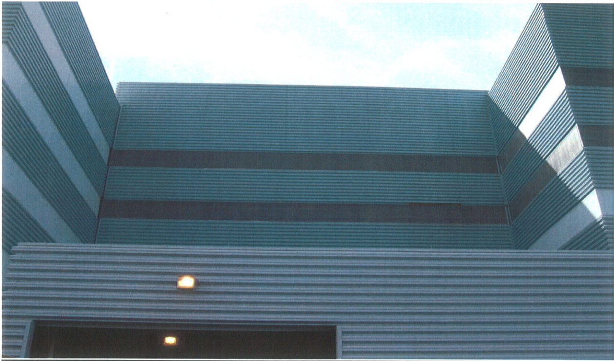
Exhibit 3 North Wall of Facility / Location of Expansion
