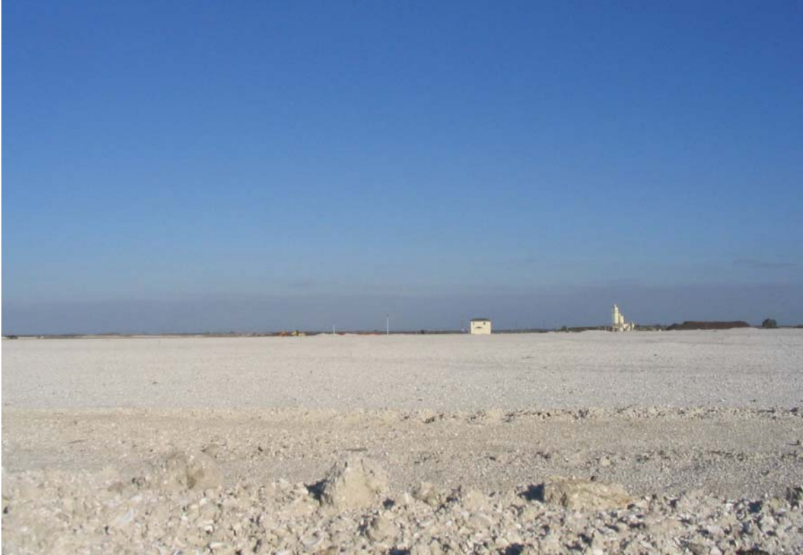
Photo 3. West County Energy Center Project Site – open land cleared of vegetation, filled, and graded.
