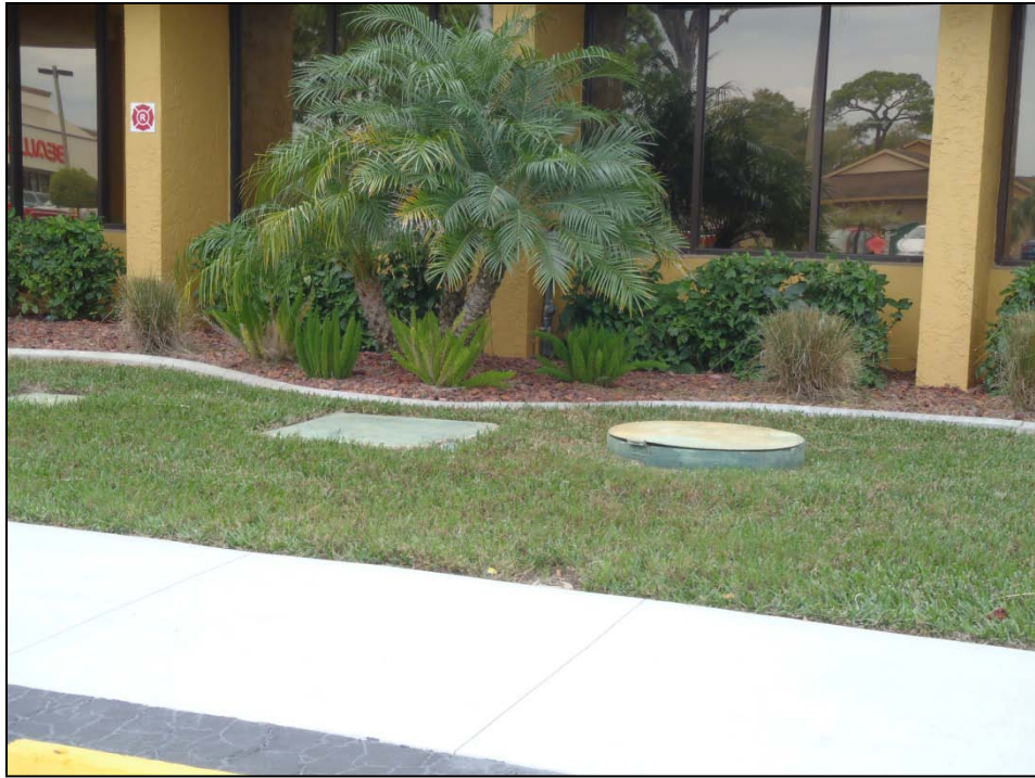
Private Lift Station P-61; Provision Eye Center 473 S. Indiana Avenue; No Emergency Signage; No Lock
