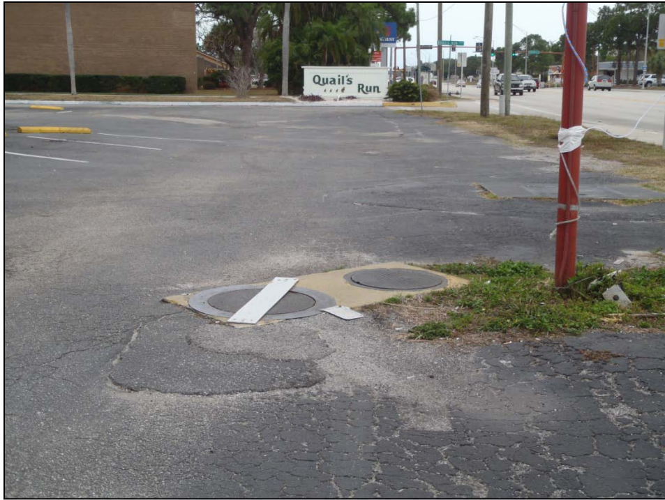
Private Lift Station P-1; Englewood Bowl 299 S. Indiana Avenue In front parking lot; No Emergency Signage or Alarm
