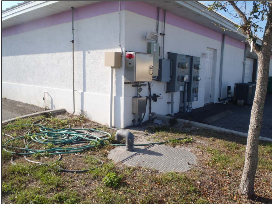
Private Lift Station P-67; Storage Units 916 S. River Rd.; No Emergency Signage
