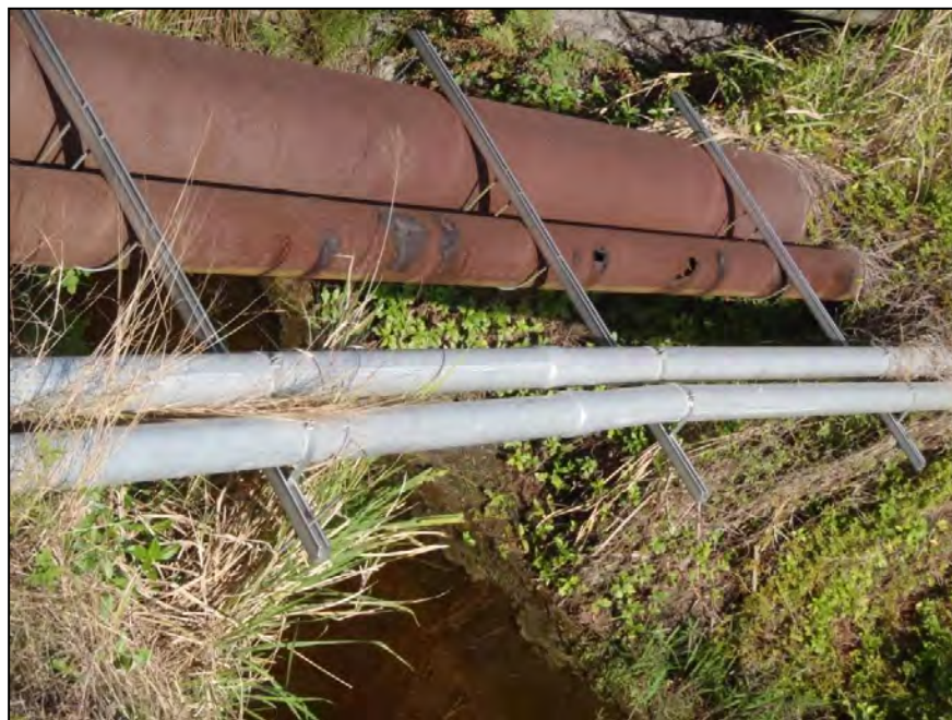
Figure 7. Aerial Crossing – Rusted out old raw water lines across open stormwater canal.
