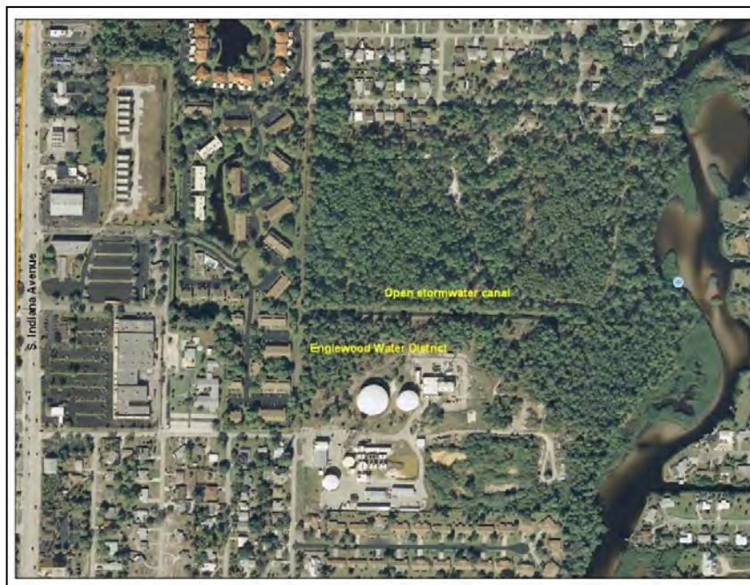
Figure 5. Open Stormwater Canal, 201 Selma Avenue – Aerial View.
