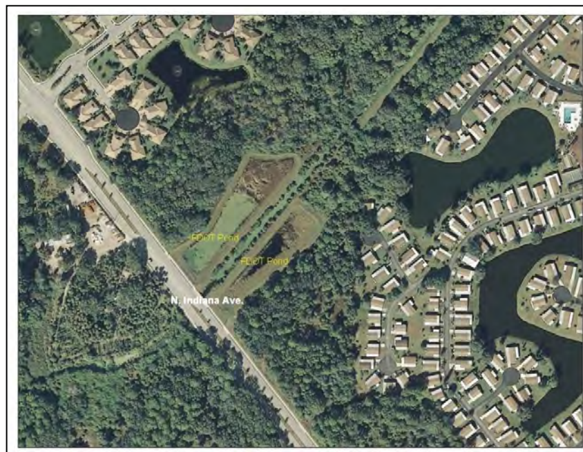
Figure 8. FDOT Stormwater Ponds.
