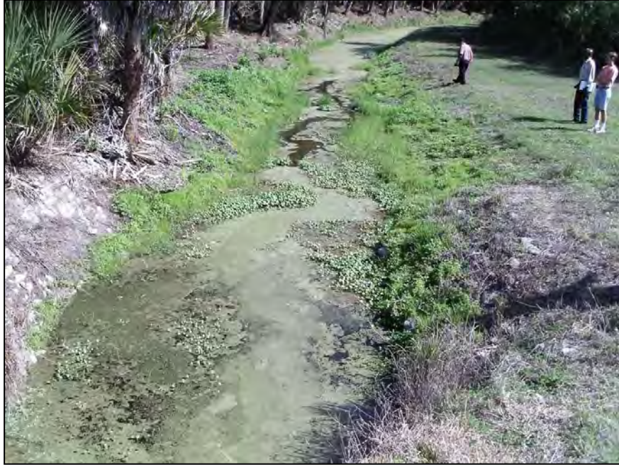
Figure 11. Englewood Lateral at Tangerine Woods Boulevard – Downstream.
