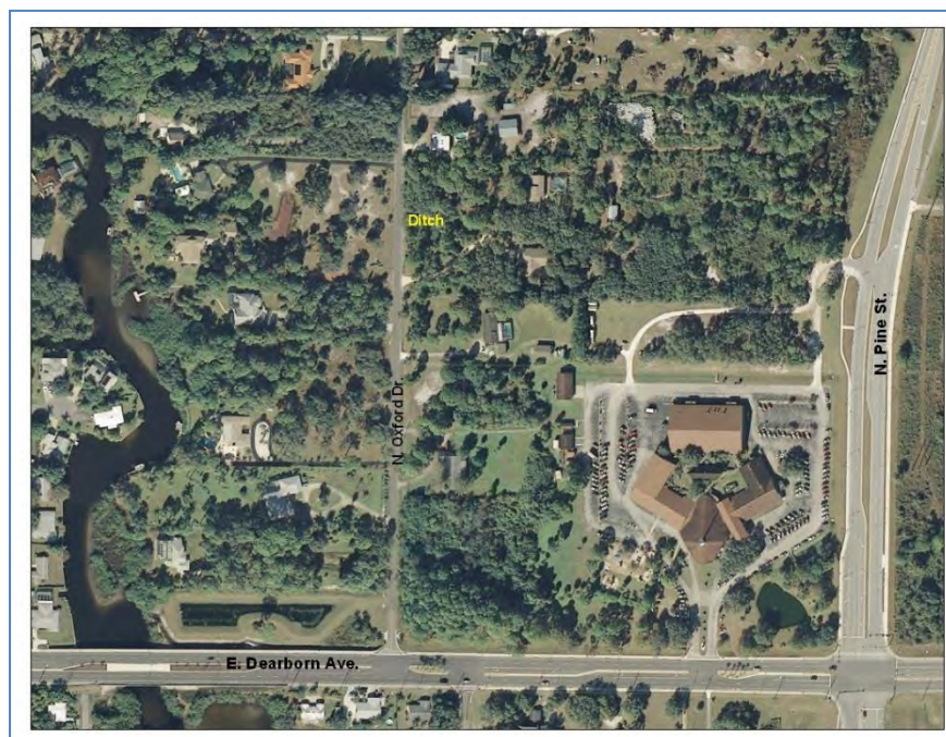
Figure 51. North Oxford Stormwater Ditch-Aerial View.
