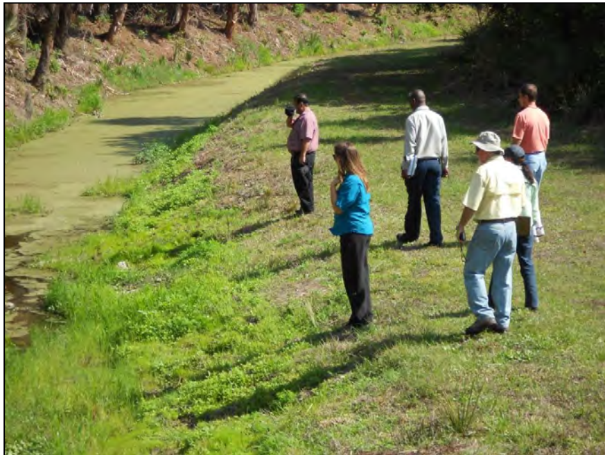
Figure 12. WTW Team Inspecting Englewood Lateral.
