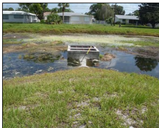
Pond Outlet Structure
