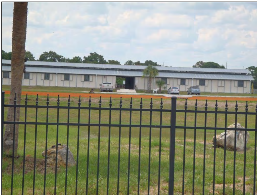
Figure 88. Crestwood Stables Barn.
