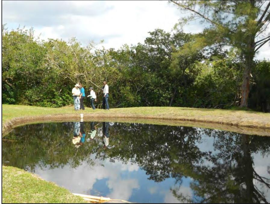
WTW Team Inspecting Berm Around Pond.
