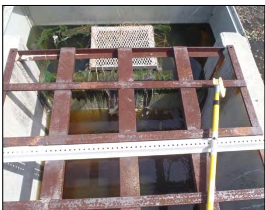
Pond outlet structure. Sample Site GOT-17
