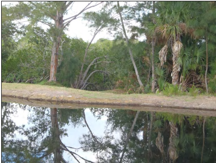
Pond Overflows Berm Directly to Creek.
