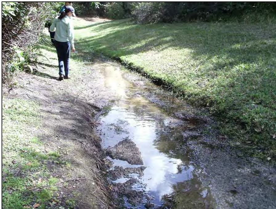
Figure 18. Foxwood Stormwater Ditch – View Toward Downstream.
