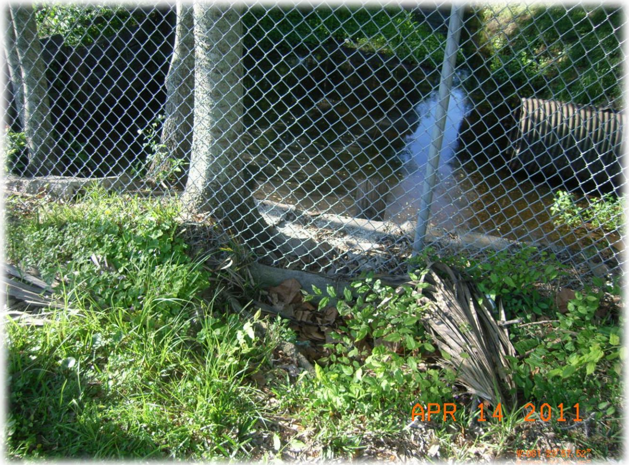
Figure 25. Point 41: Jacksonville Beach at 15 th Ave. N. (FDOT ditch).
