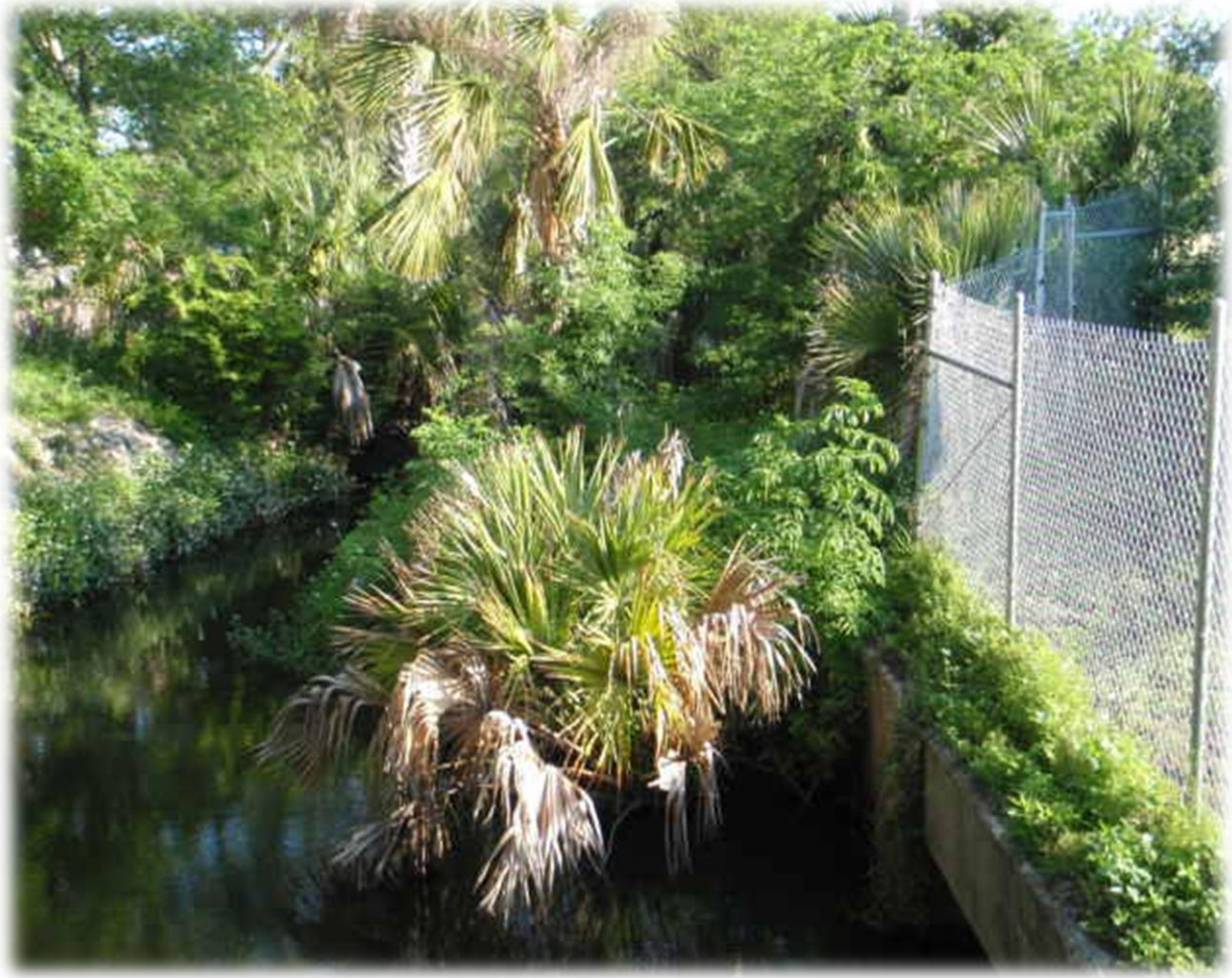
Figure 27. Point 41: Jacksonville Beach at 15th Ave. N. (FDOT ditch).
