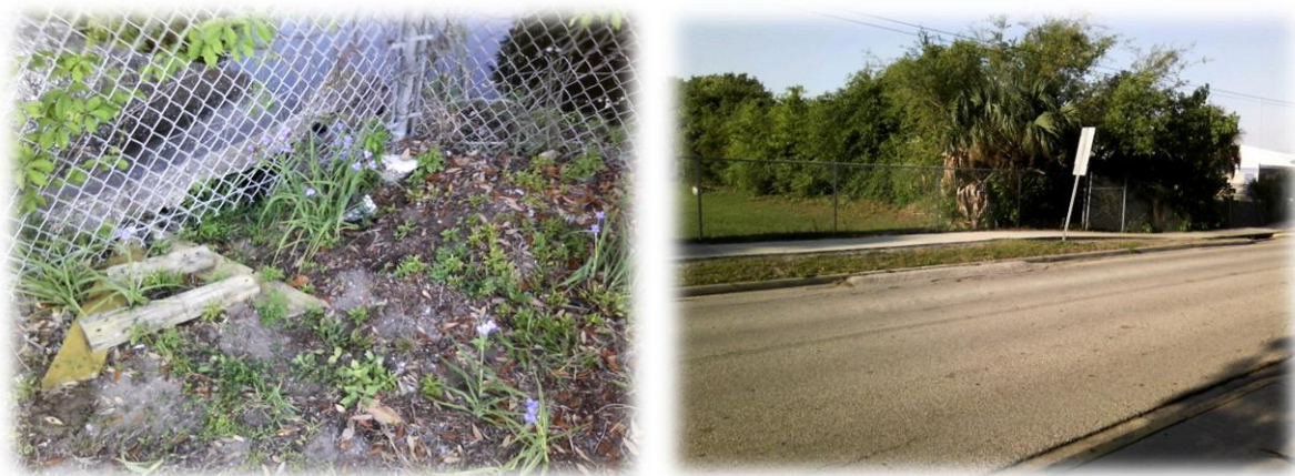
Figure 18. Point 35: Border of Jacksonville and Neptune Beach, FDOT ditch at Seagate Ave.
