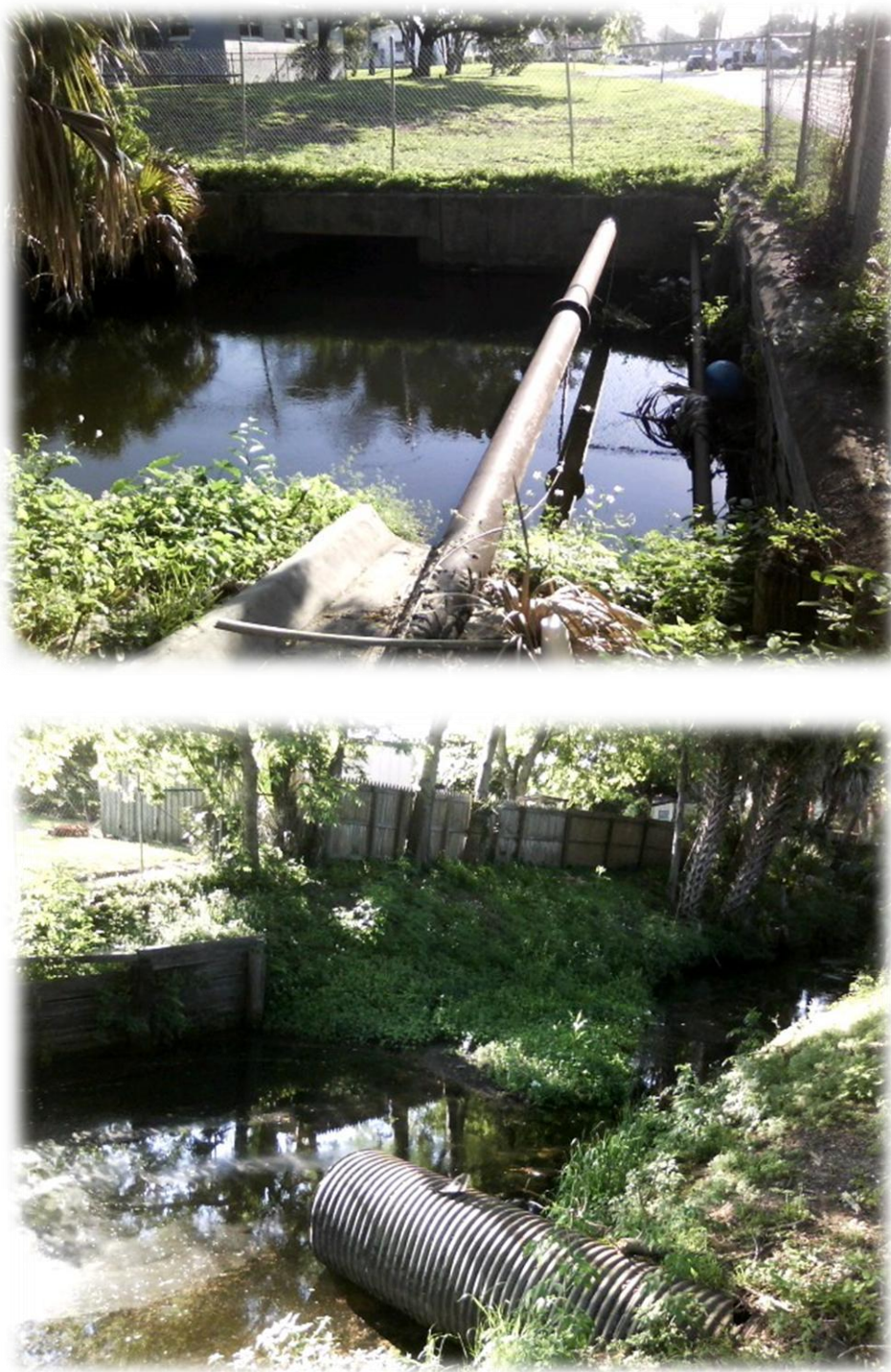
Figure 24. Point 41: Jacksonville Beach at 15 th Ave. N. (FDOT ditch).
