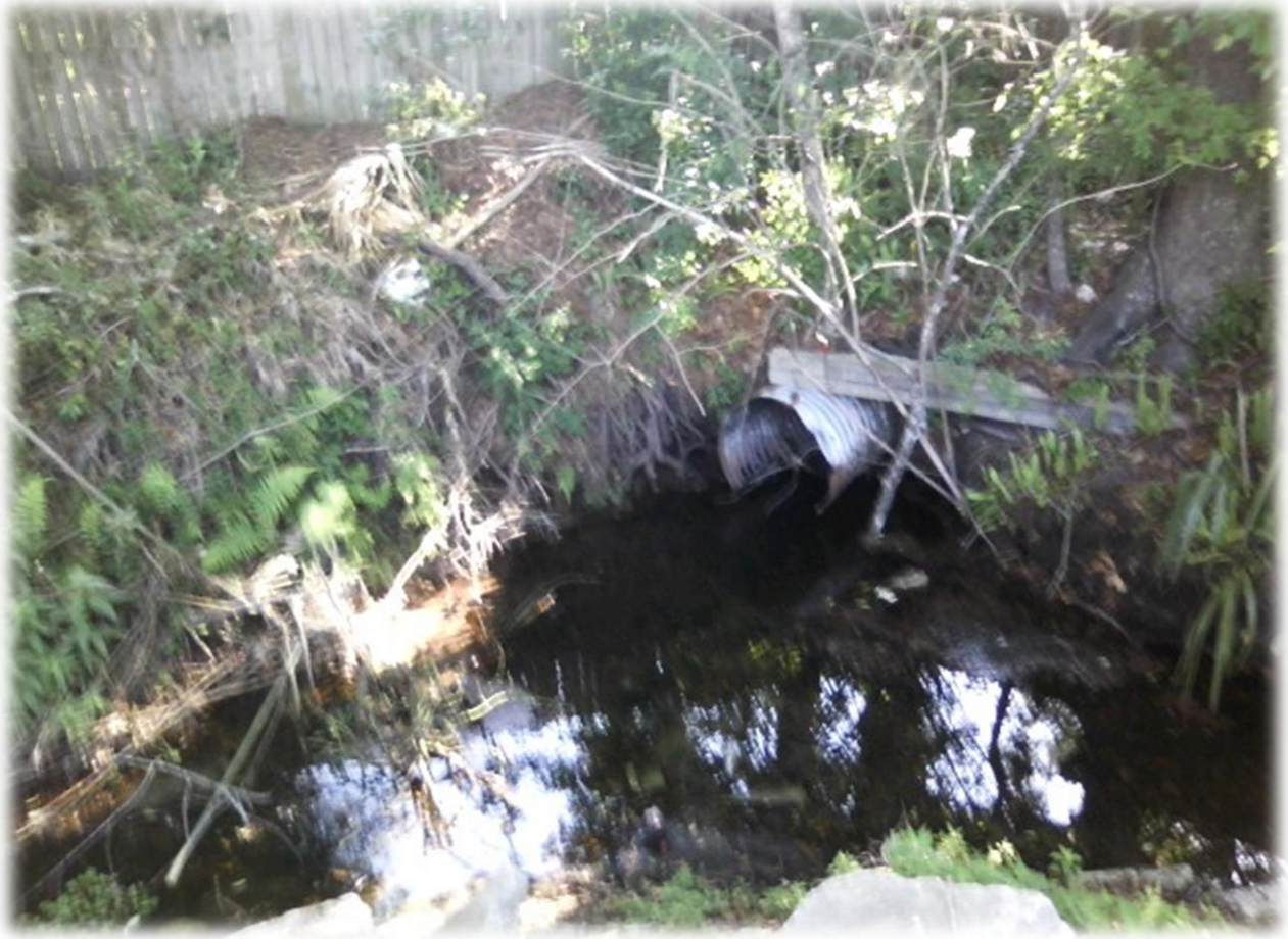
Figure 31. Jacksonville Beach, just downstream of Point 59.
