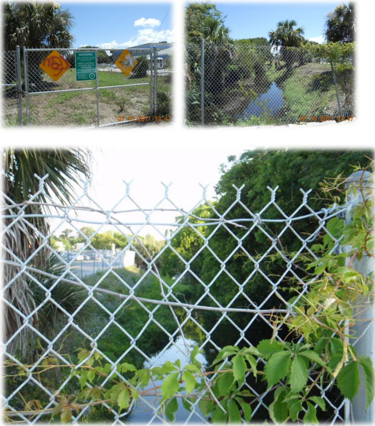
Figure 20. Point 35: Border of Jacksonville and Neptune Beach, FDOT ditch at Seagate Ave.
