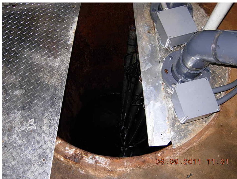
Figure 55. Views of the second VA Hospital sanitary lift station, also located inside one of the buildings. A noticeable sewage odor with ammonia prevailed. The pump station is sealed.
