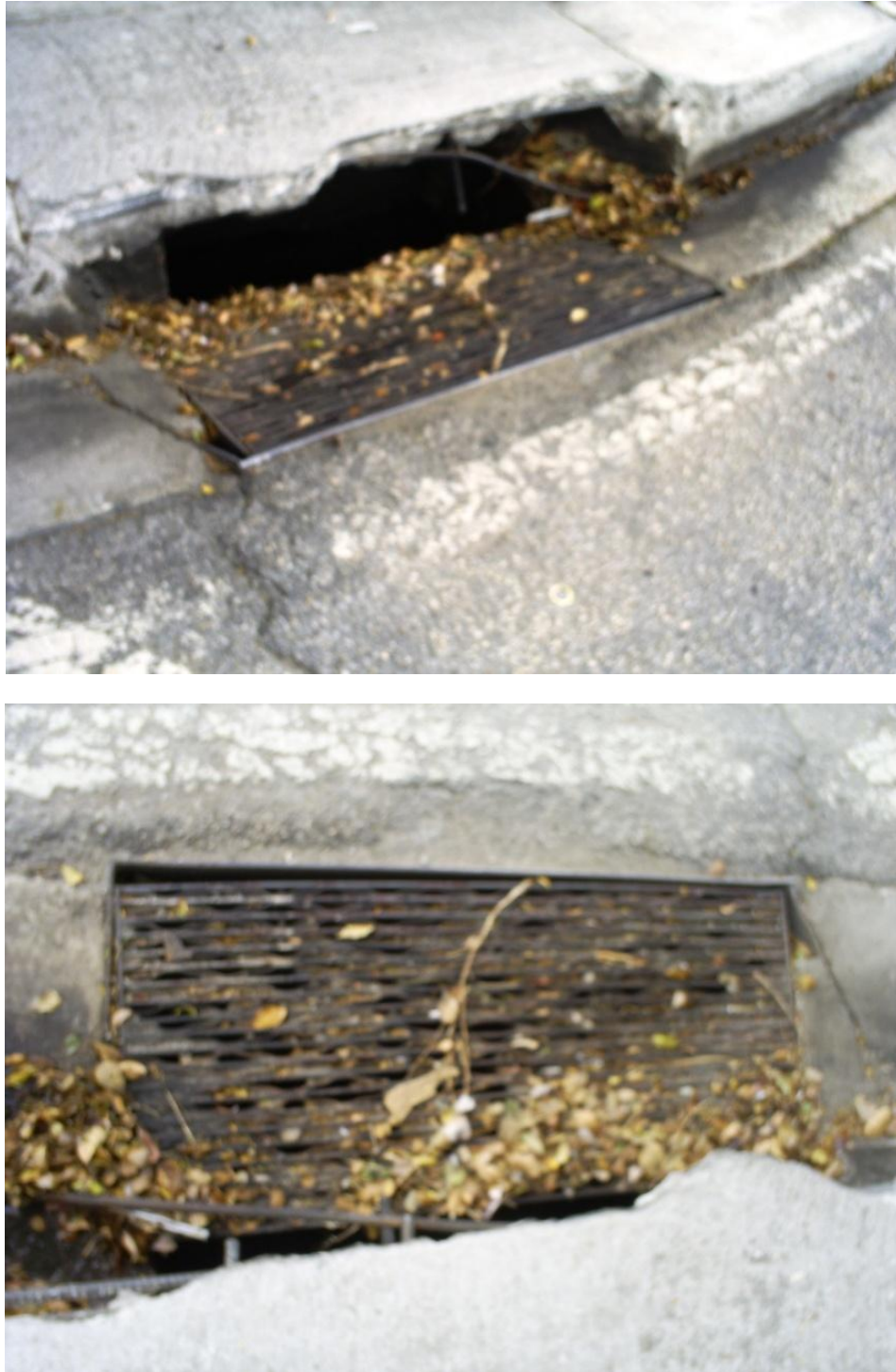
Figure 19. Broken storm drain covers at NW 20 th Street belonging to Miami-Dade County; the openings allow trash and other materials to enter the underground conveyance directly and provide a breeding ground for fecal coliform.
