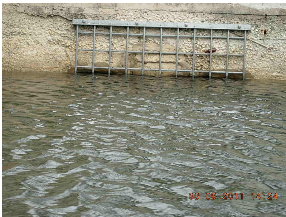
Figure 74. A sealed outfall with a manatee grate at NW 7 th Avenue and NW 7 th Street. No GPS coordinates were taken.
