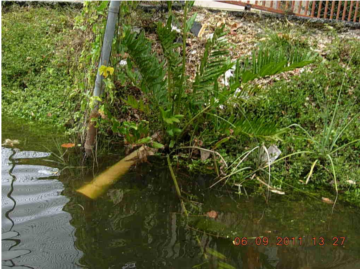
Figure 67. A polyvinyl chloride (PVC) pipe approximately 2 inches in diameter located near the southern boundary of the property could be a PIC or an irrigation line. GPS coordinates are 25 47' 35.028" N, 80 13' 13.741" W.
