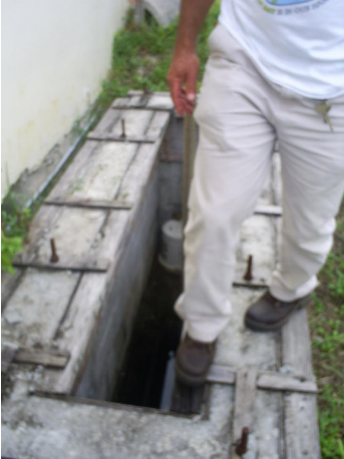
Figure 46. A PIC at the City of Miami Overtown stormwater pump station consists of those portions of the incomplete upgrades that allow foreign objects to enter the stormwater system.
