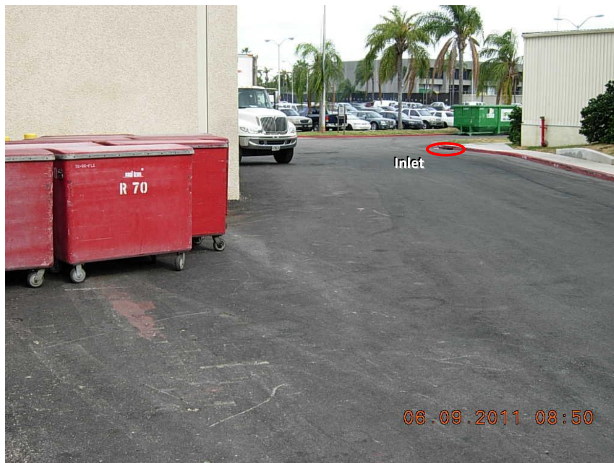
Figure 53. View of a portion of the VA Hospital site, near the western parking lot. On the way in to inspect the sanitary lift stations, the team observed closed biomedical waste bins upstream of the curb opening inlet (circled in red at top right). One of the team members observed some small holes in the bins. In the same area, a roll-off container was observed upslope of a drop inlet (at left).
