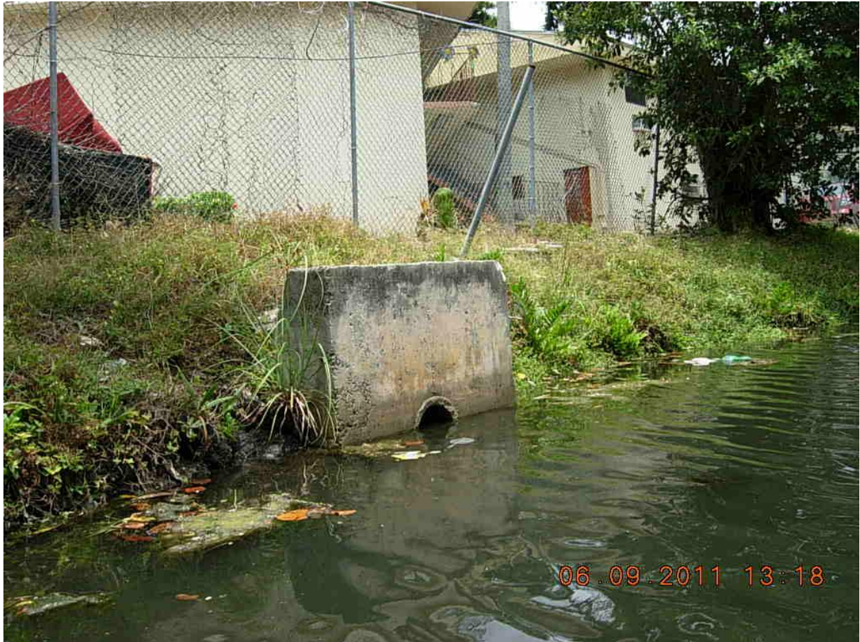
Figure 63. The first PIC was an 8-inch-diameter concrete pipe with a headwall. GPS coordinates are 25 47' 37.142" N, 80 13' 15.892" W.
