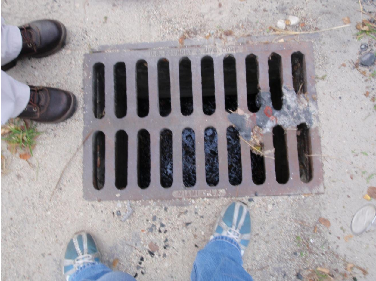
Figure 20. A storm drain on NW 15 th Avenue south of NW 20 th Street is filled with trash and not draining properly; any flooding that results could cause a failure of the wastewater system, and trash can provide a breeding ground for fecal coliform.
