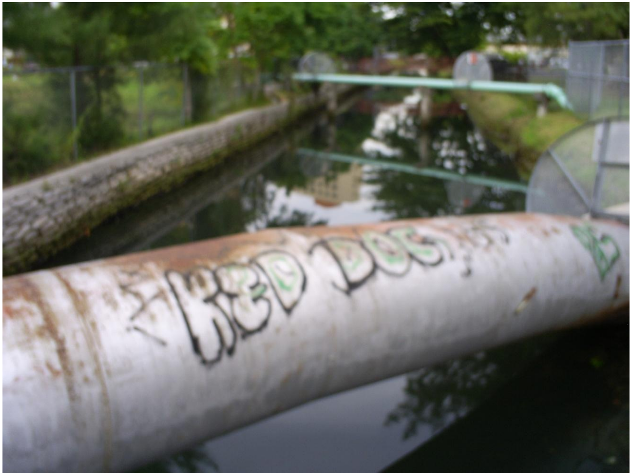
Figure 39. Abandoned sewer line crossing the creek north of the NW 17 th Street Bridge.
