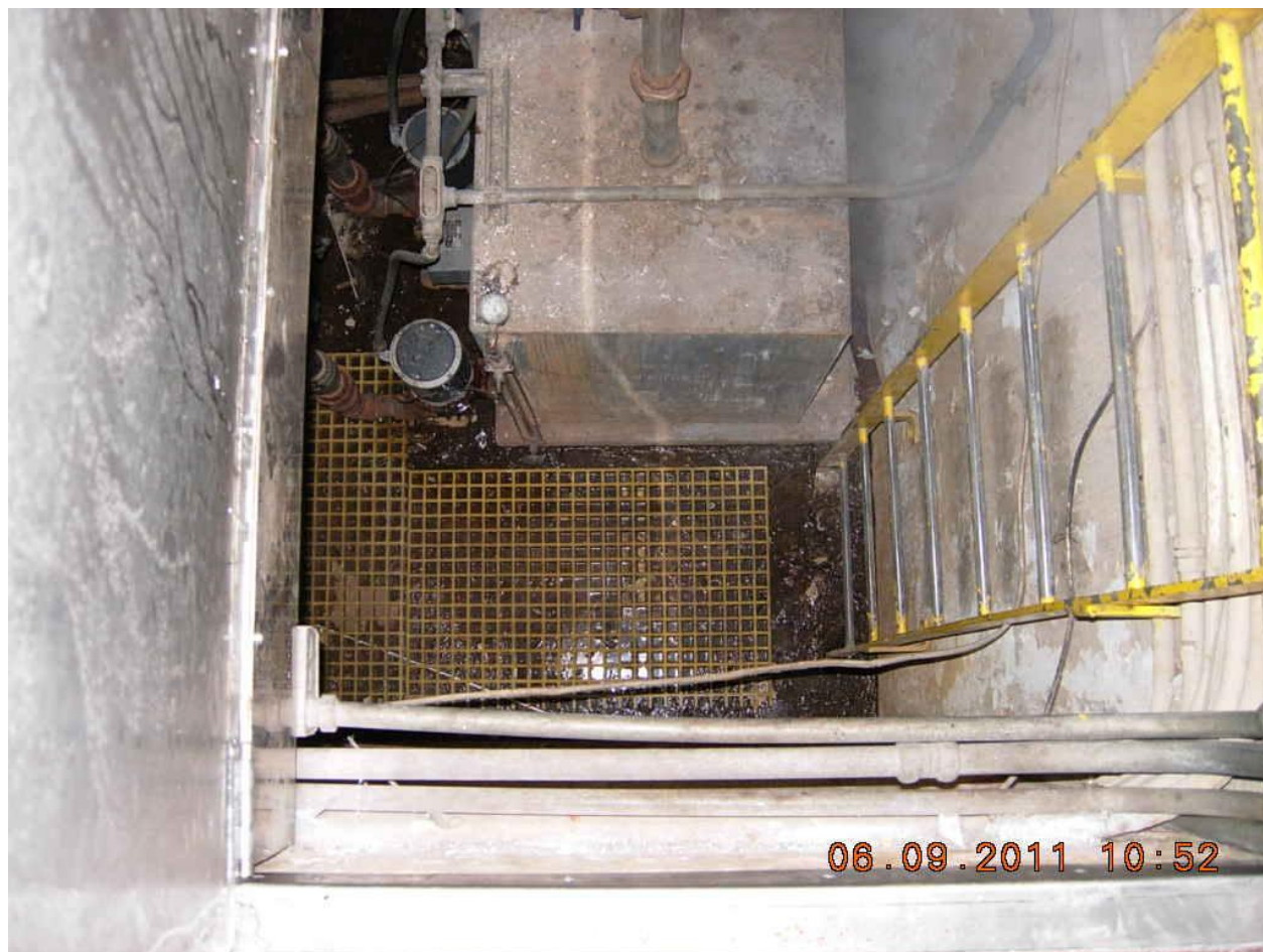
Figure 54. View of the first VA Hospital sanitary lift station, located inside one of the buildings. The VA staff stated that the pump station was “open” rather than “sealed” because it is located in an area where there is a continuous flow of air from outside. Harold Moesch from FDEP entered the pump station for a closer investigation. No unusual conditions were observed. There was a noticeable mercaptan odor at this location.
