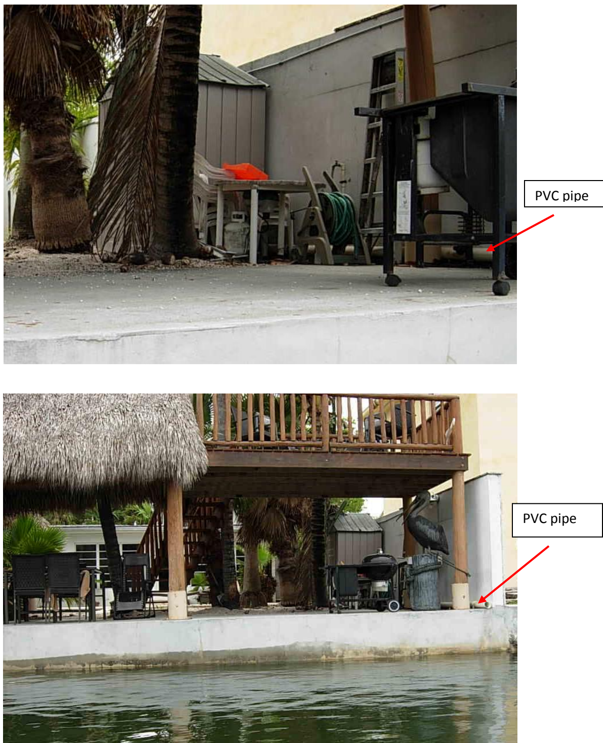
Figure 81. At 727 NW 7 th Street, the team observed a 4-inch white PVC pipe running from the property line at Seybold Canal towards the front of the property.
