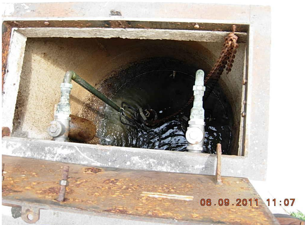
Figure 56. Views of the VA Hospital sanitary lift station located outside between Buildings 8 and 9. The pump station appeared relatively clean. No grease was observed.
