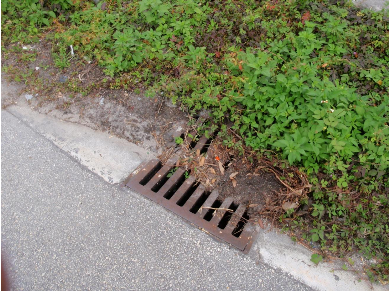
Figure 25. View of a partially blocked stormwater drain at 1501 to 1511 NW 13 th Court; any flooding that results could lead to the failure of septic and wastewater infrastructure.
