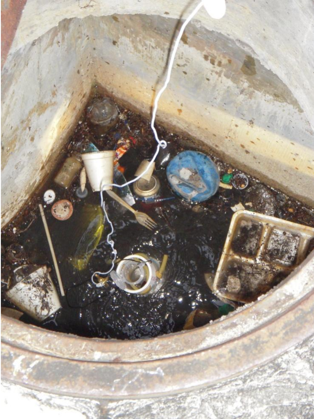
Figure 3. Trash and debris in a stormwater manhole thought to be at the headwaters.
