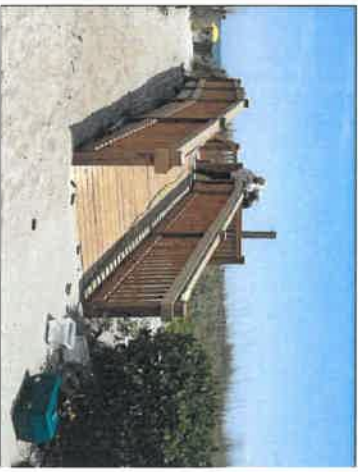
VEGETATION AVOIDANCE OPTION 2 – TYP TIMBER DUNE WALKOVER STRUCTURE
