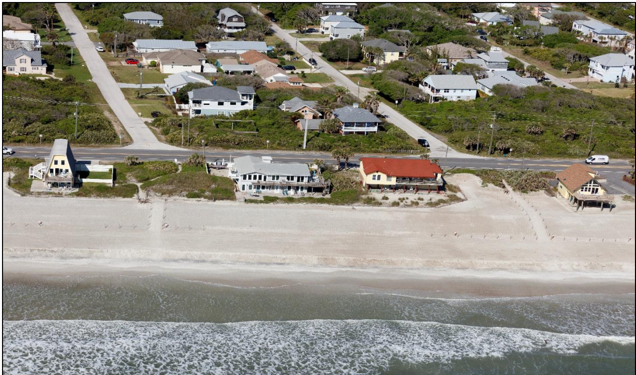
Figure D-14. Post-Construction Condition near T-110 (Apr. 2021)
