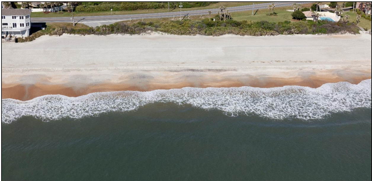
Figure D-2. Post-Construction Condition near T-104 (Apr. 2021)
