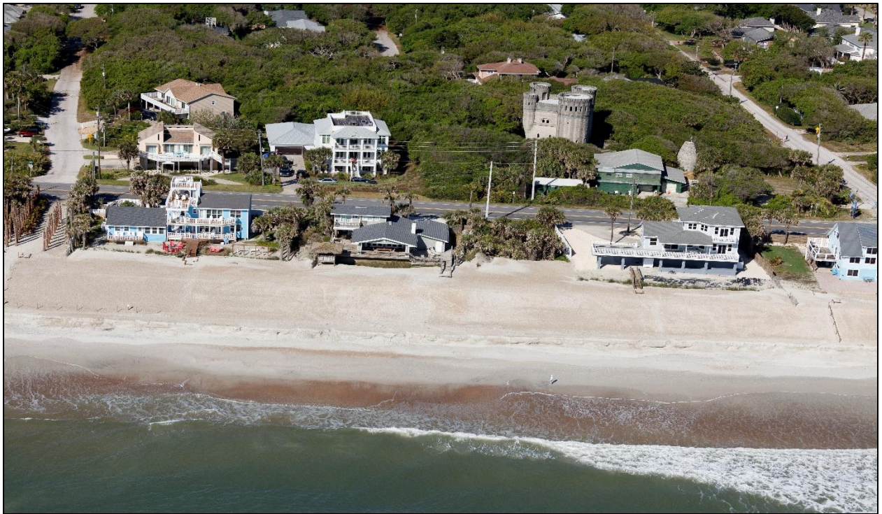
Figure D-10. Post-Construction Condition near R-108 (Apr. 2021)
