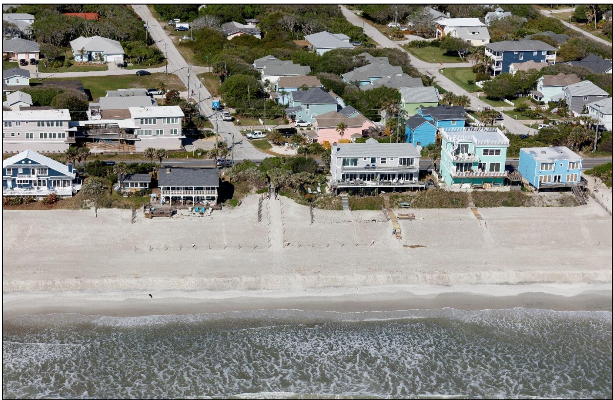
Figure D-16. Post-Construction Condition near R-111 (Apr. 2021)
