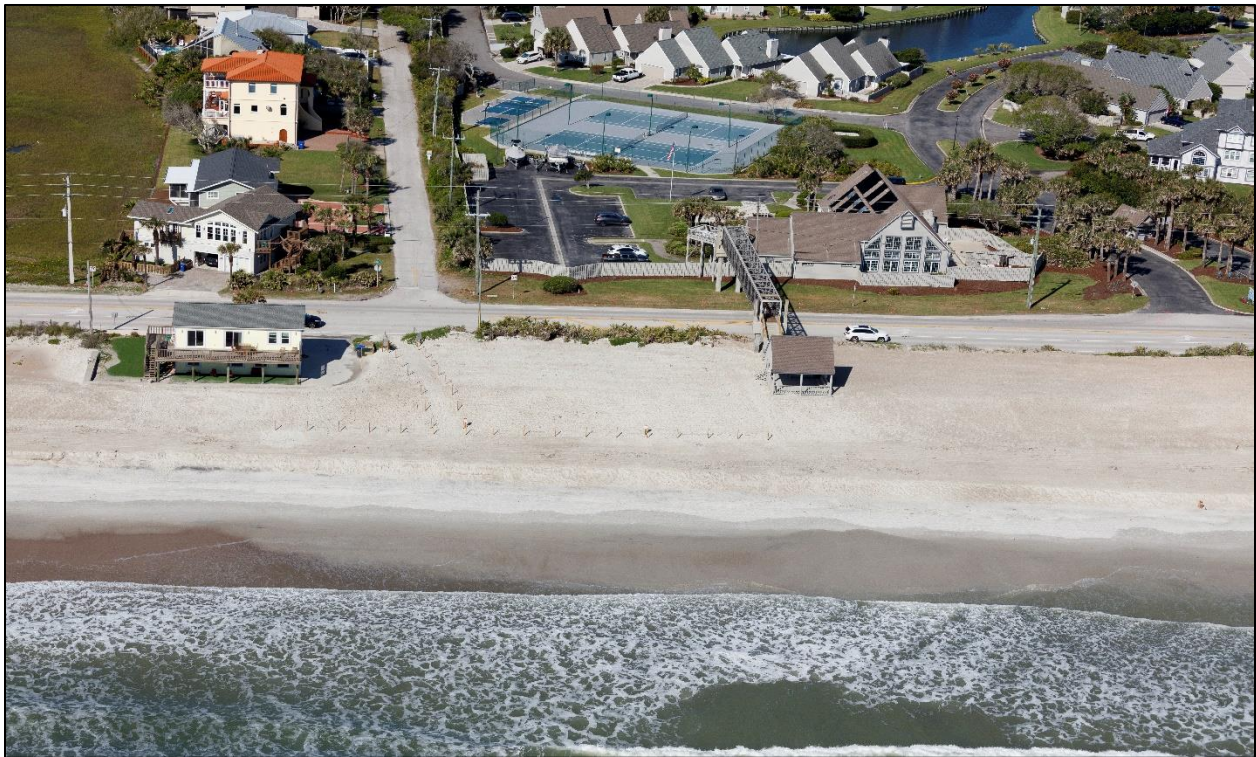
Figure D-22. Post-Construction Condition near T-114 (Apr. 2021)
