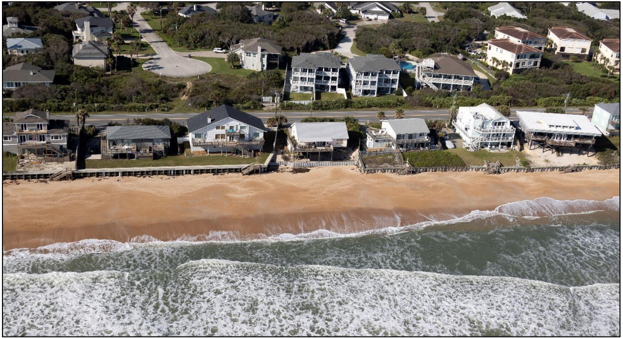
Figure D-7. Pre-Construction Condition near R-107 (Nov. 2020)
