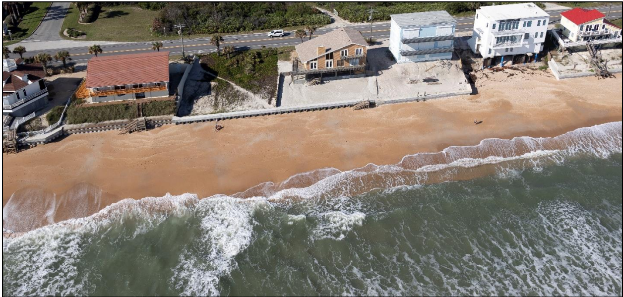
Figure D-5. Pre-Construction Condition near R-106 (Nov. 2020)
