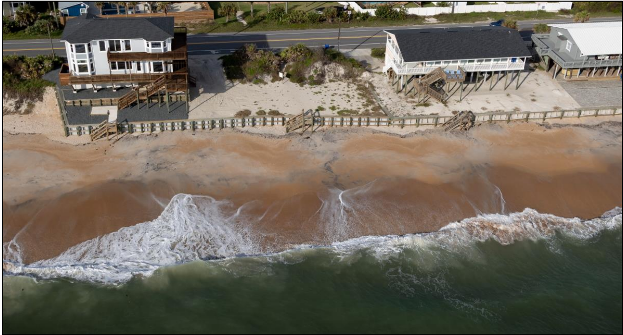
Figure D-17. Pre-Construction Condition near T-112 (Oct. 2020)
