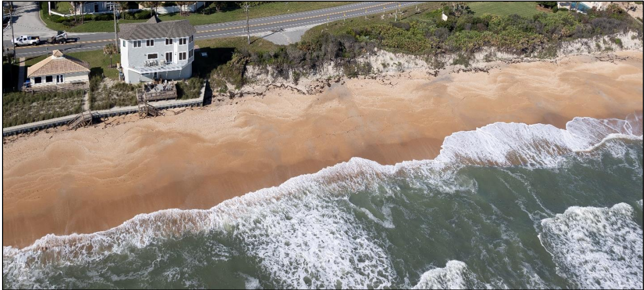
Figure D-1. Pre-Construction Condition near T-104 (Nov. 2020)
