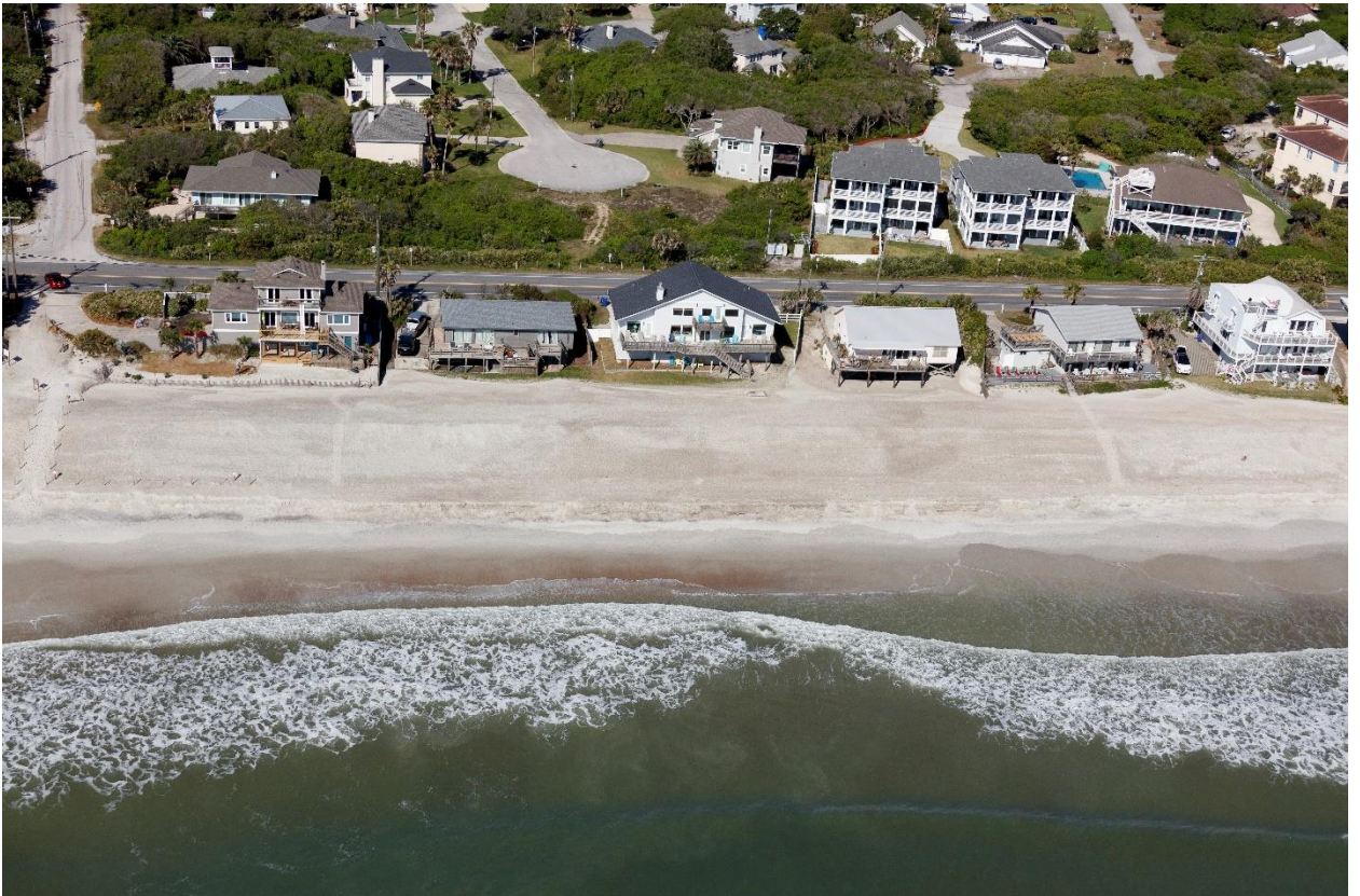
Figure D-8. Post-Construction Condition near R-107 (Apr. 2021)
