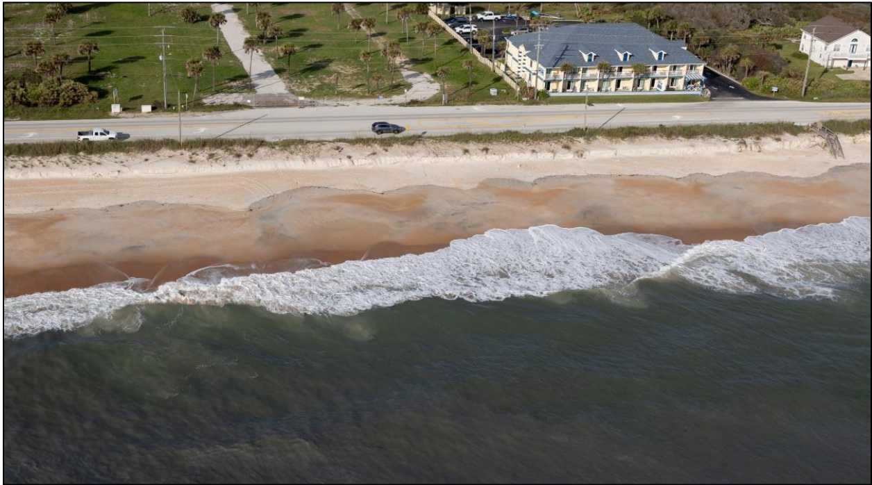
Figure D-23. Pre-Construction Condition near R-115 (Oct. 2020)
