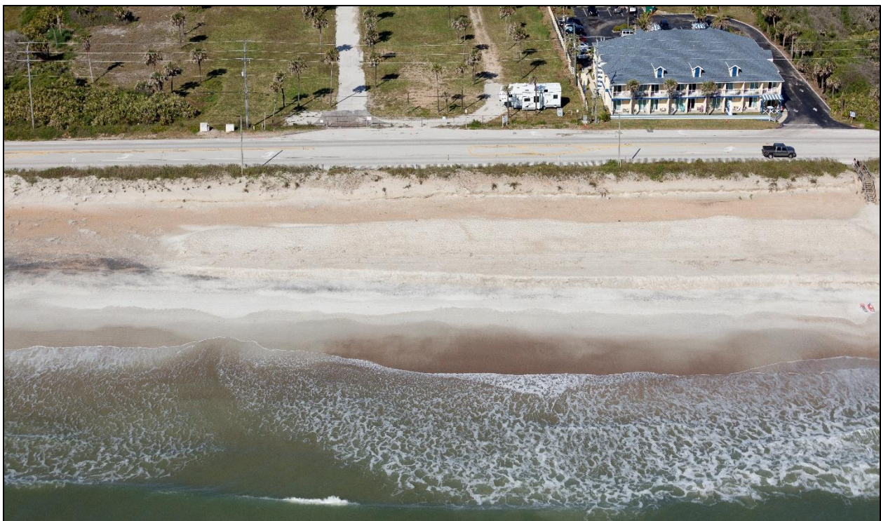
Figure D-24. Post-Construction Condition near R-115 (Apr. 2021)
