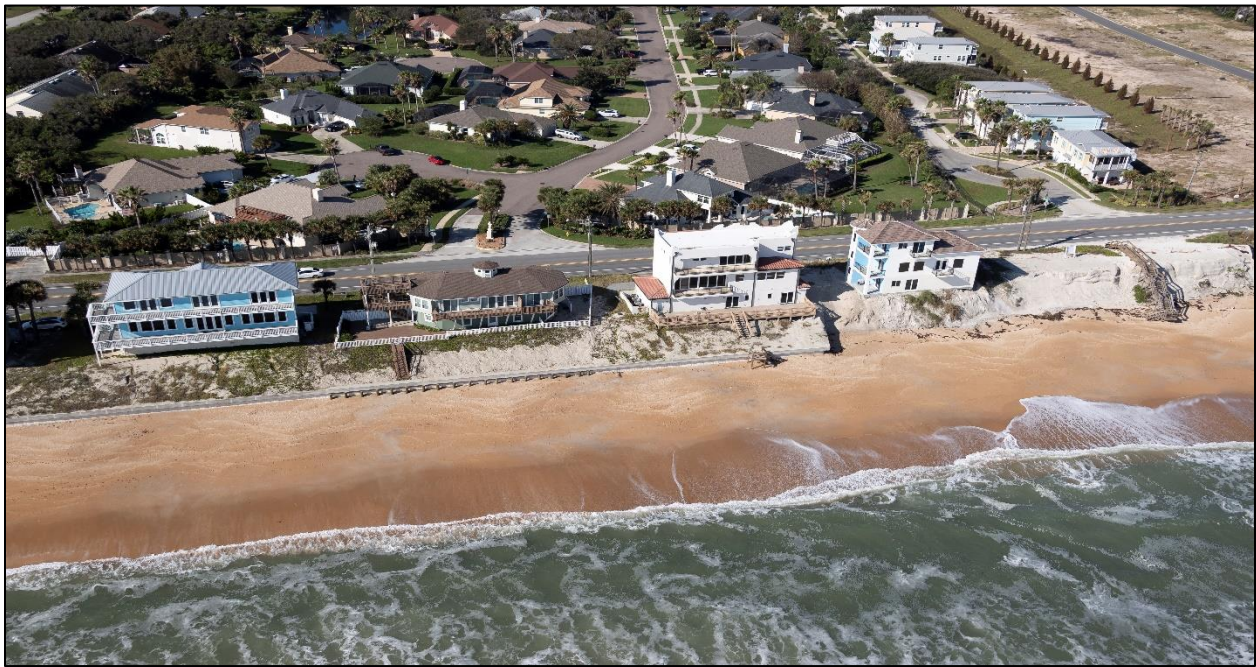
Figure D-3. Pre-Construction Condition near R-105 (Nov. 2020)
