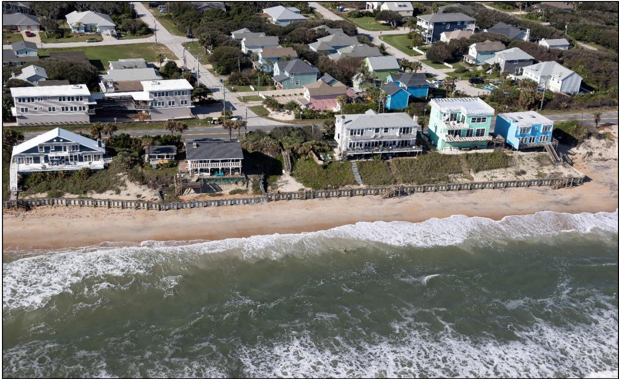
Figure D-15. Pre-Construction Condition near R-111 (Nov. 2020)
