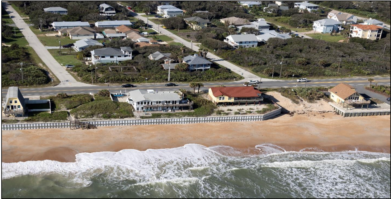
Figure D-13. Pre-Construction Condition near T-110 (Nov. 2020)
