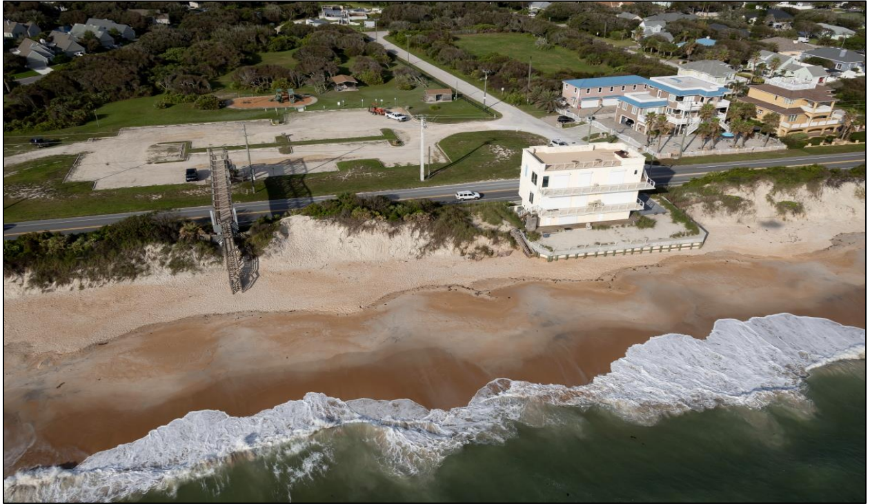
Figure D-19. Pre-Construction Condition near R-113 (Oct. 2020)
