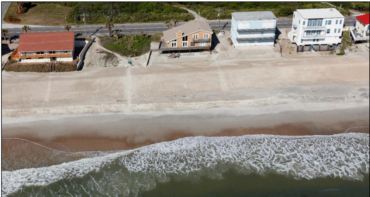
Figure D-6. Post-Construction Condition near R-106 (Apr. 2021)
