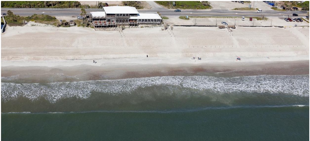
Figure D-12. Post-Construction Condition near R-109 (Apr. 2021)
