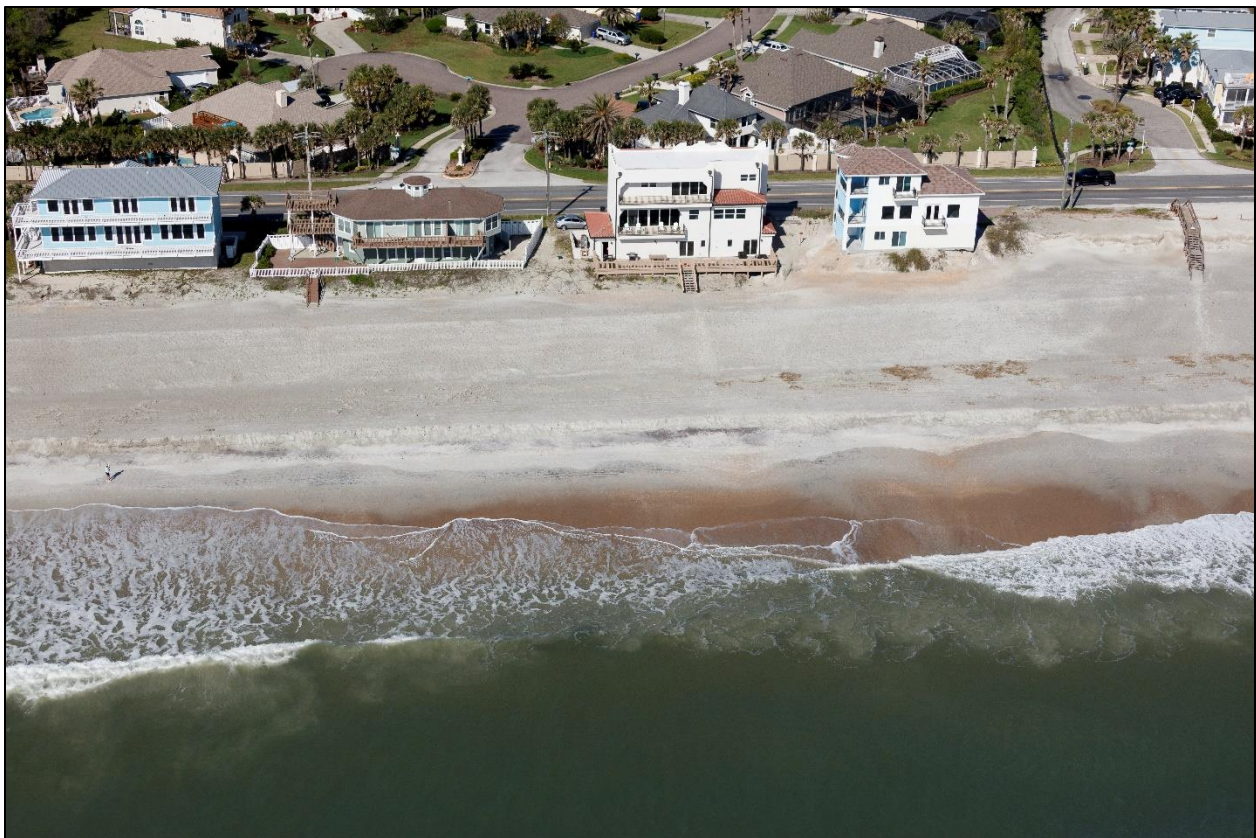
Figure D-4. Post-Construction Condition near R-105 (Apr. 2021)
