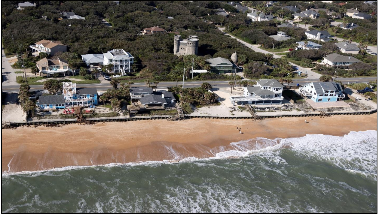
Figure D-9. Pre-Construction Condition near R-108 (Nov. 2020)
