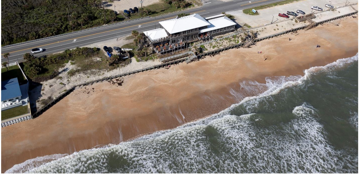
Figure D-11. Pre-Construction Condition near R-109 (Nov. 2020)
