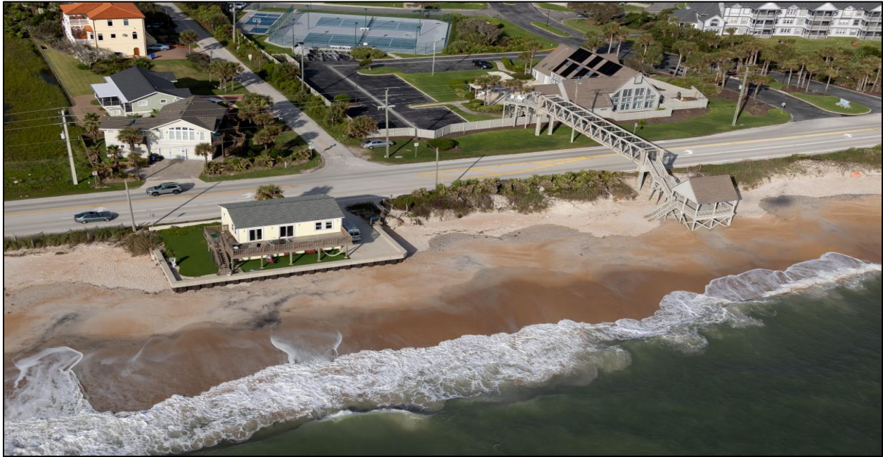
Figure D-21. Pre-Construction Condition near T-114 (Oct. 2020)
