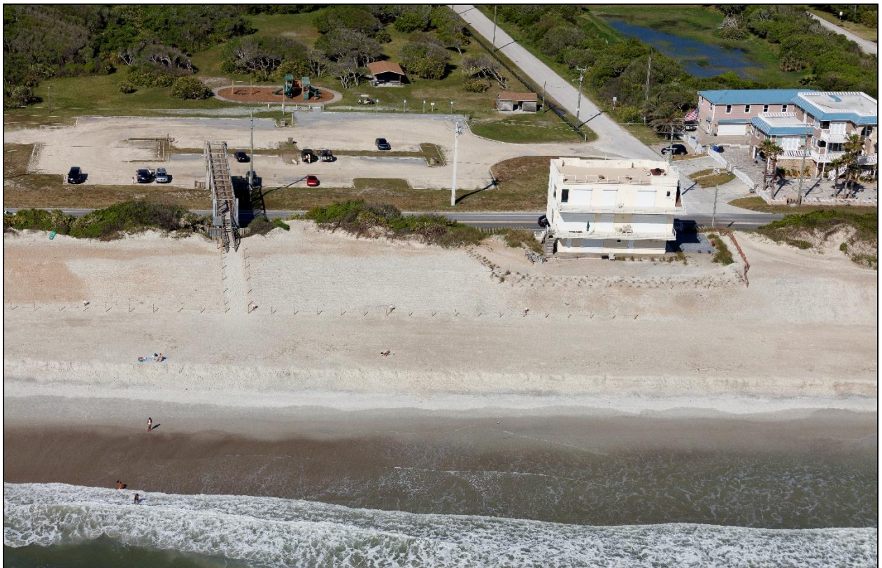
Figure D-20. Post-Construction Condition near R-113 (Apr. 2021)
