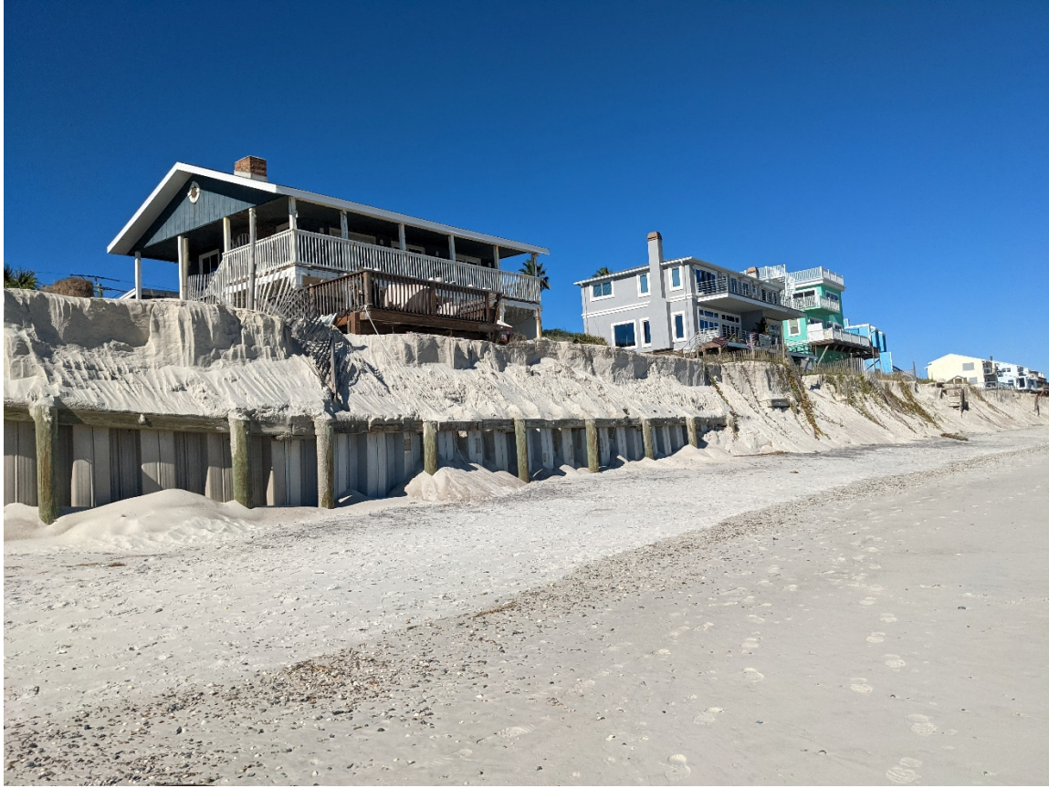
Figure 3: Photo facing northwest just south of Boating Club Road (just south of R-109) showing post-storm dune scarping, exposure of pre-existing seawalls, and undermining of beach access structures. November 16, 2021
