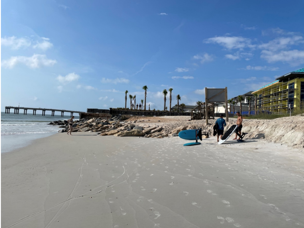
Figure D.35: St Johns County R-141 looking South (07/23/21)
