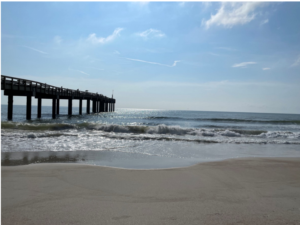
Figure D.38: St Johns County R-142 looking East (07/23/21)
