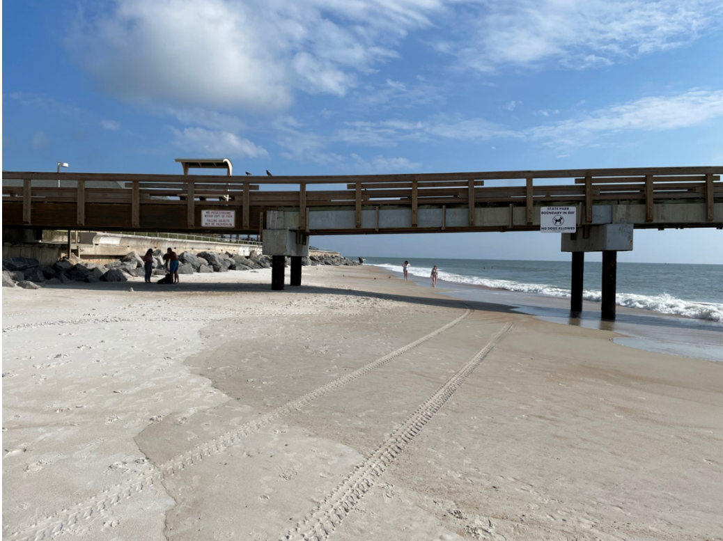
Figure D.37: St Johns County R-142 looking North (07/23/21)
