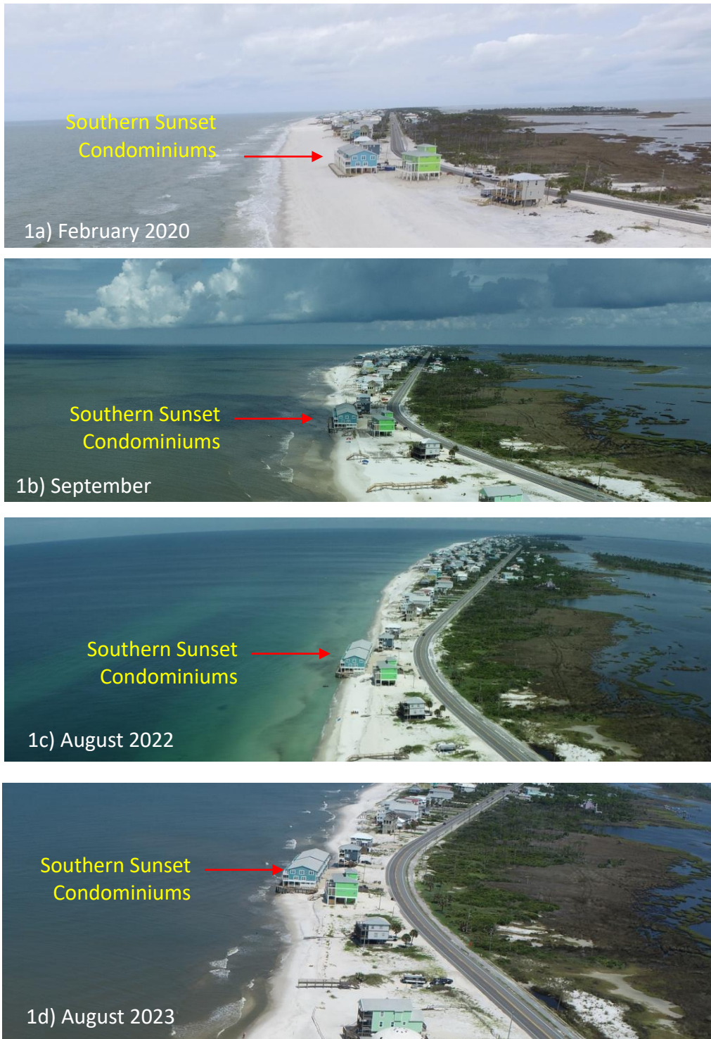
Photo 1 (a-d.) Shoreline evolution in the vicinity of the Southern Sunset Condominiums in (a) February 2020 (post-construction), (b) September 2021, (c) August 2022, and (d) August 2023 looking from south to north.
