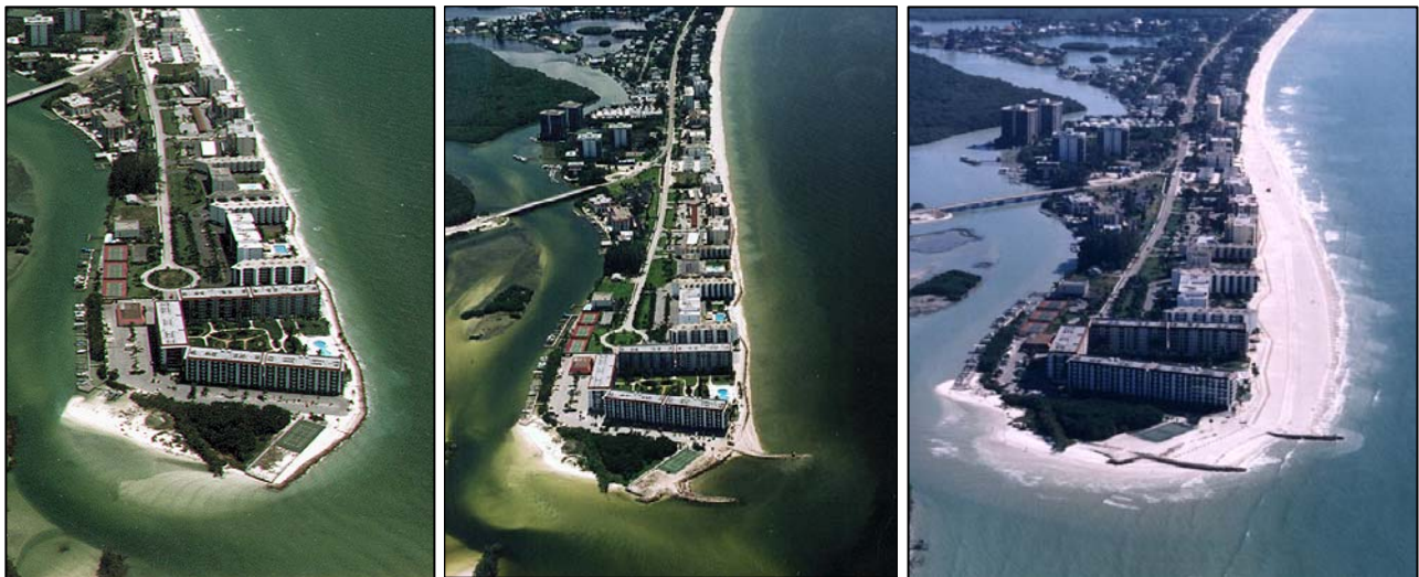
Figure 1: North end of Bonita Beach before construction of the terminal groins (left), after construction of the terminal groins (middle), and after placement of 217,000 cy of sand 1 (right).
