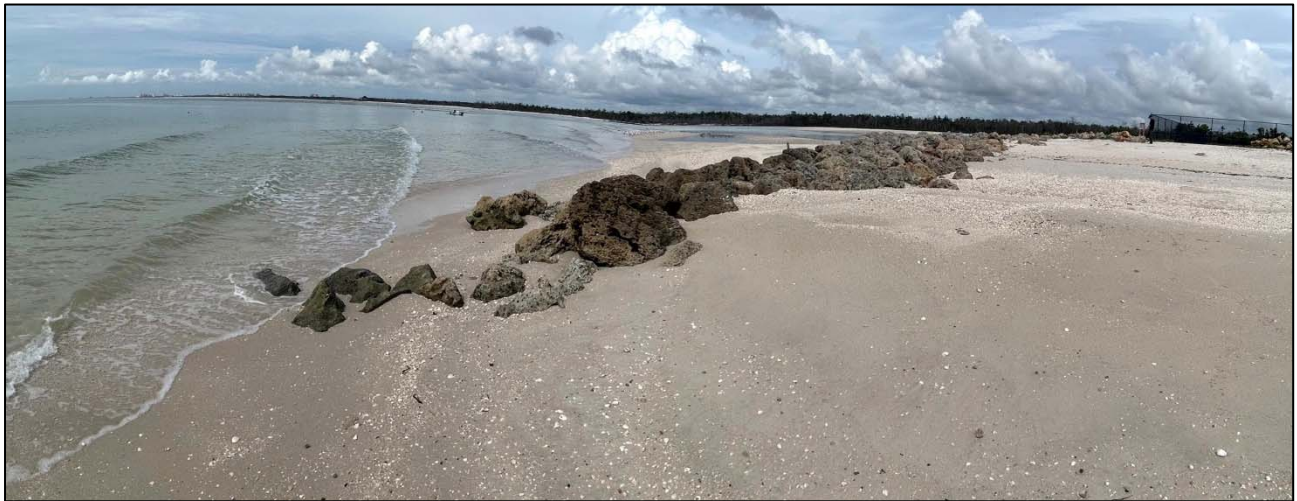
North Groin – Seaward End (9/26/2023).
