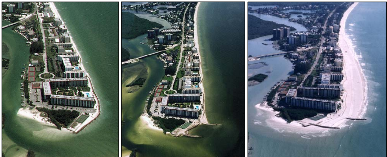
Figure 1: North end of Bonita Beach before construction of the terminal groins ( left ), after construction of the terminal groins ( middle ), and after placement of 217,000 cy of sand 3 ( right ).
