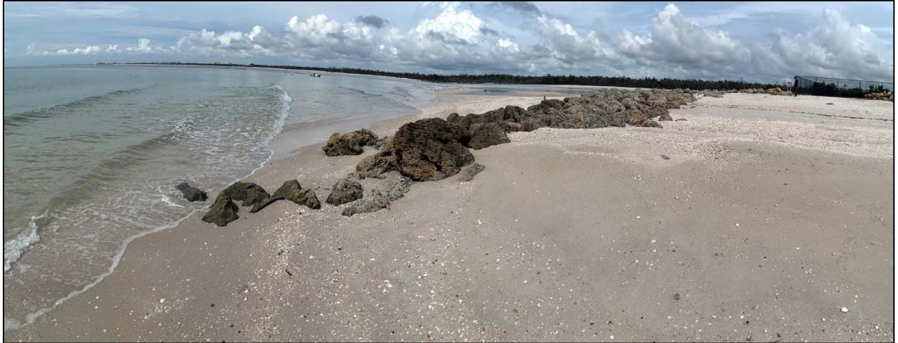
North Groin – Seaward End (9/26/2023).
