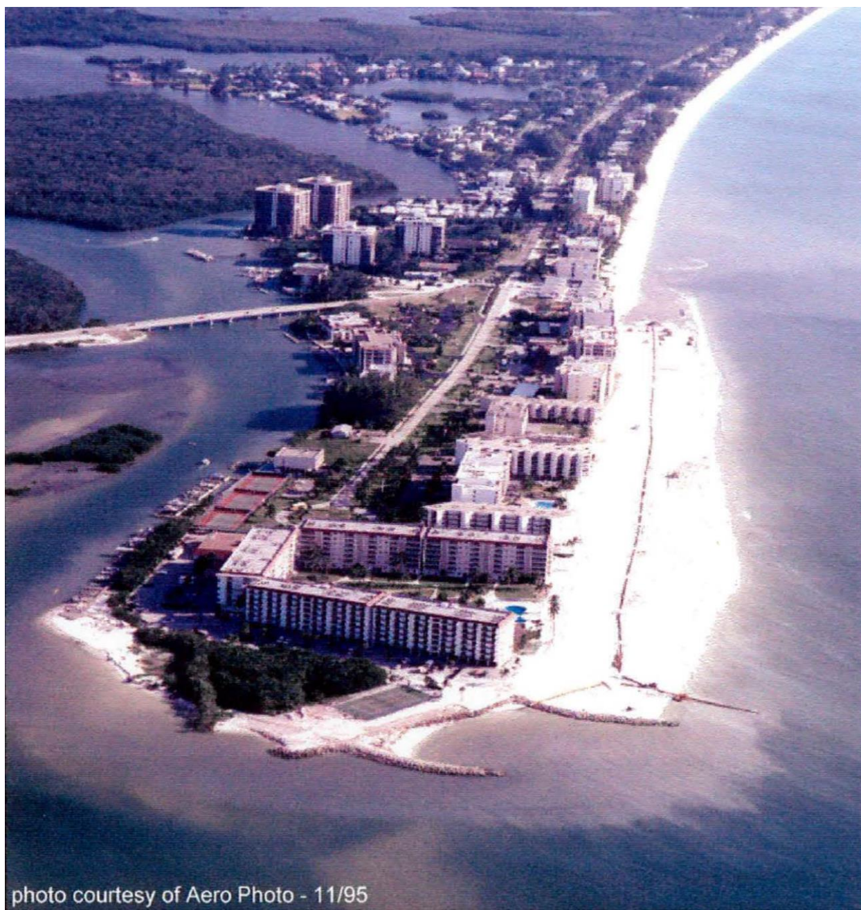
Figure 2. Photo of 1995 Construction Project (from Olsen, 1996).
