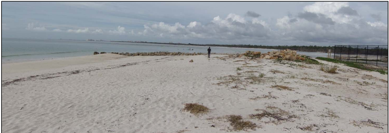
North Groin – Profile (9/26/2023), with scattered rock stockpiled along the beach berm at right. [The deposition of a low sand berm along the shoreline, evident in the photograph above, is a residual result of Hurricane Idalia in late August 2023.]
