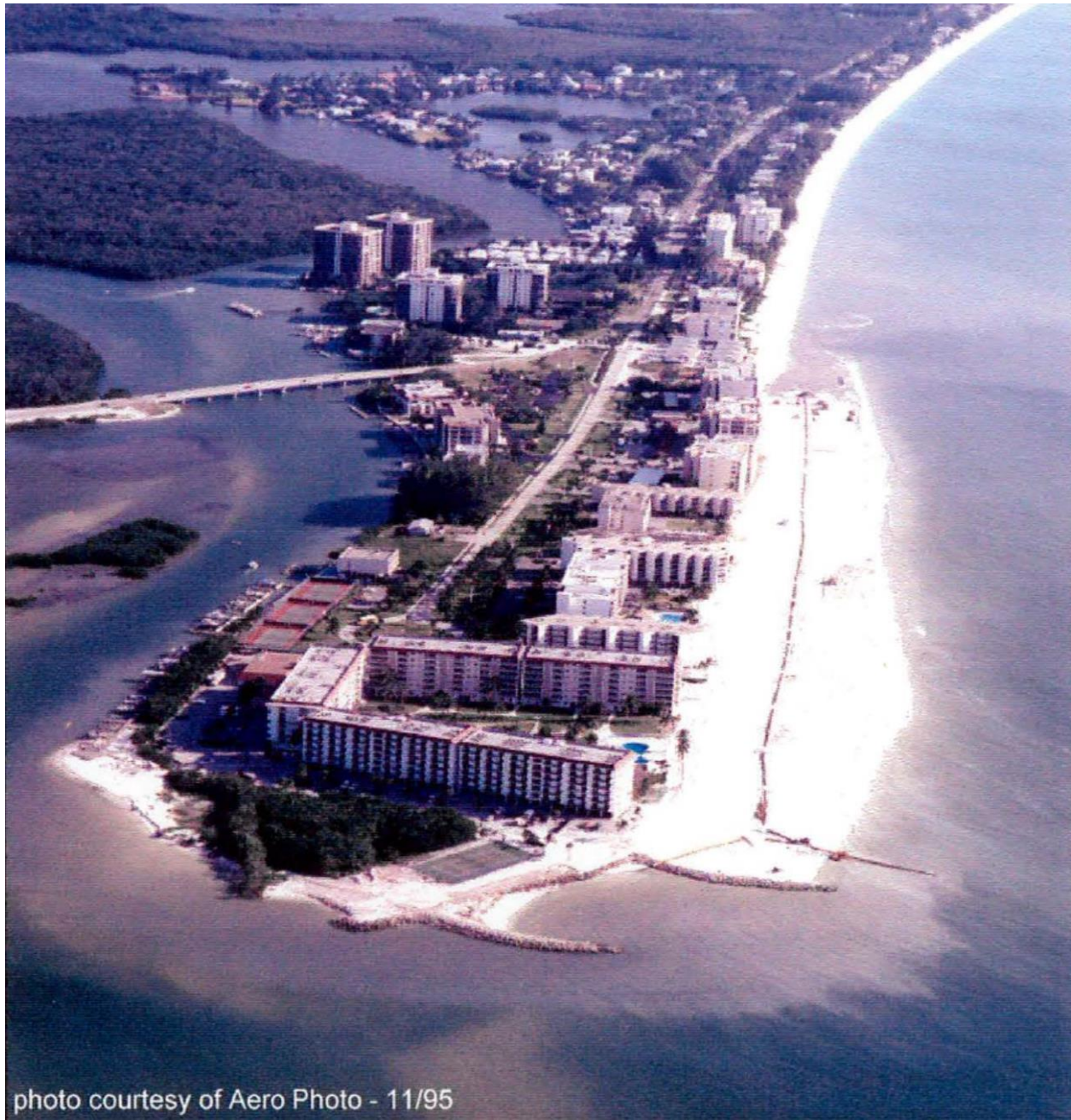
Figure 2. Photo of 1995 Construction Project (from Olsen, 1996).
