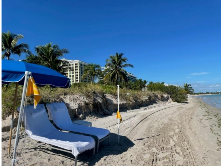
Figure 6. Escarpment observed in the vicinity of R-104.5 looking North
