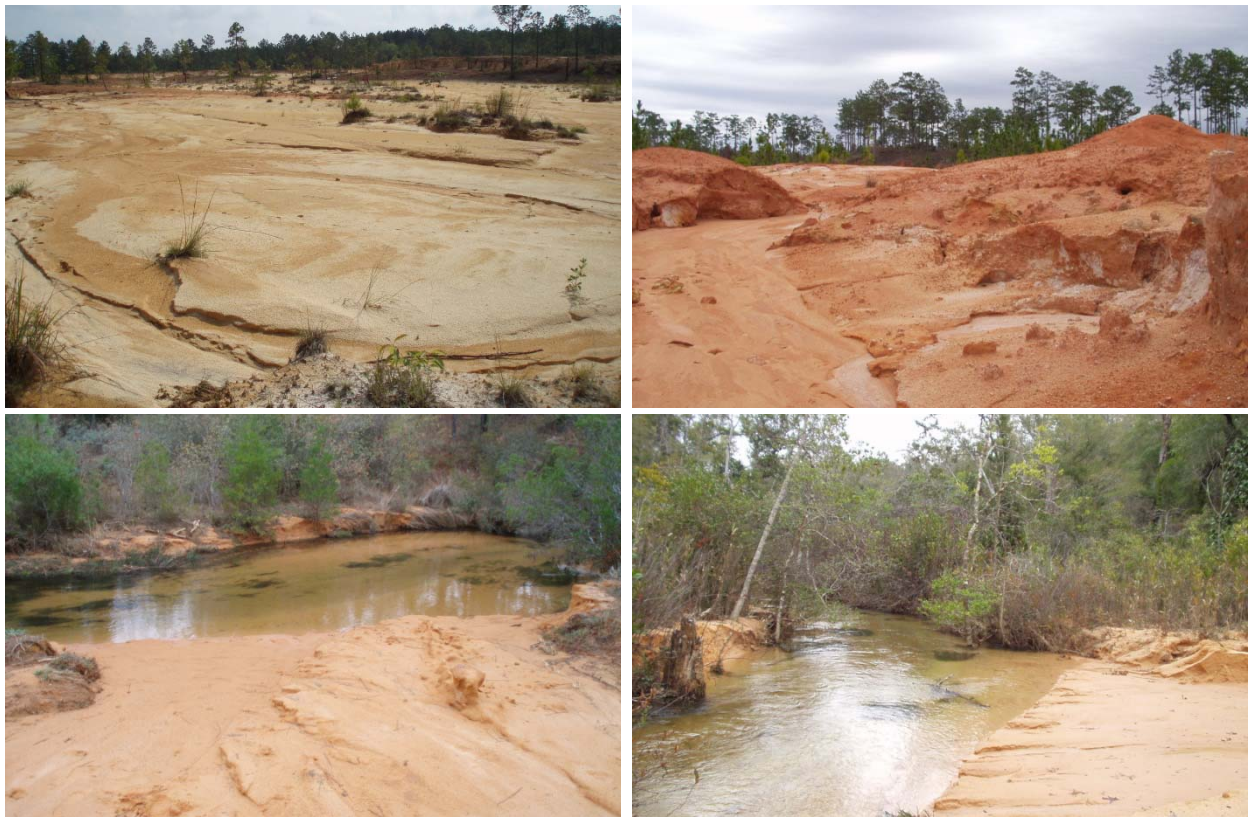
Figure 9. Examples of Northwest Florida Borrow Pit-Induced Erosion and Sedimentation
