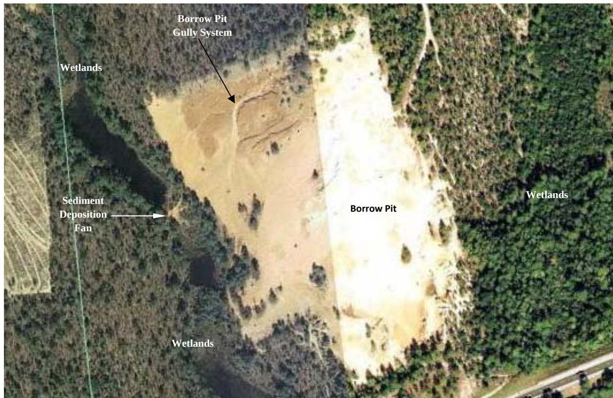
Figure 6. Northwest Florida Borrow Pit Soil Erosion and Off-Site Sediment Discharge (Google Earth)
