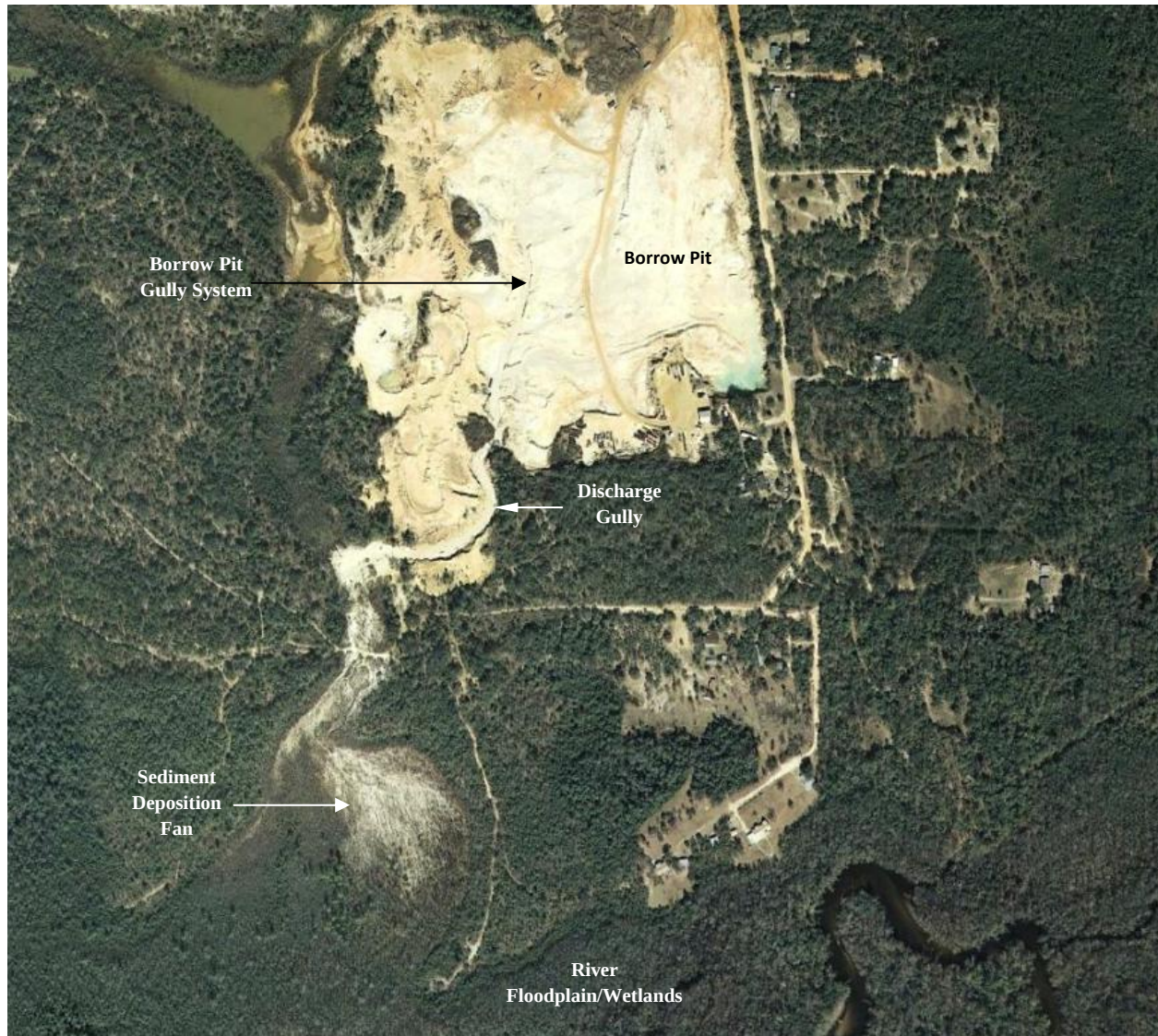
Figure 7. Northwest Florida Borrow Pit Soil Erosion and Off-Site Sediment Discharge (Google Earth)
