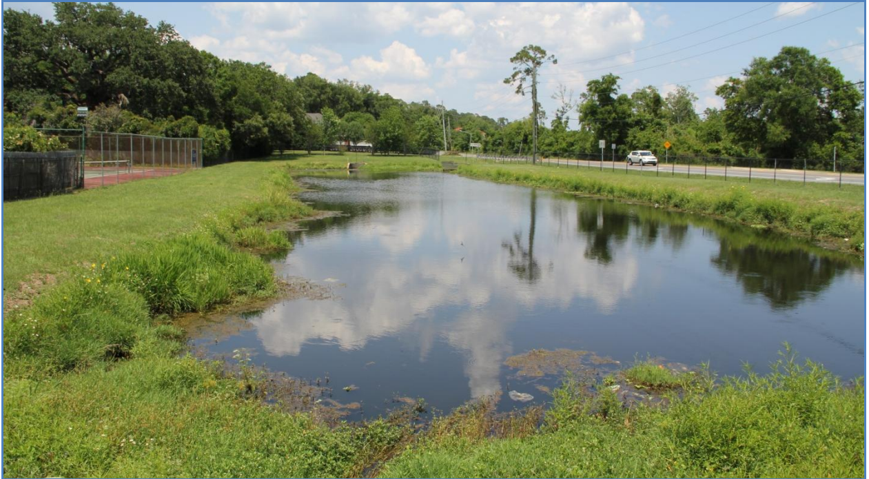
Retention pond at the corner of US 90 (Scenic Highway) and Langley Road.
