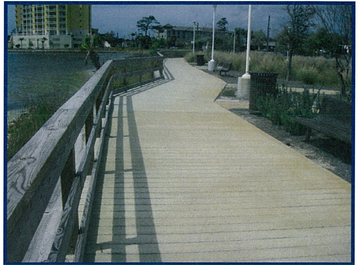
Photo 2. Existing portion of boardwalk project constructed in 2007 along Santa Rosa Sound.
