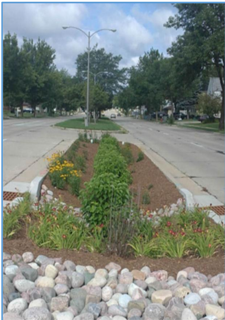
Example of a Bioswale Median
