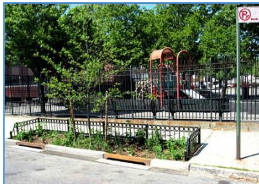
Examples of Bioswale Storm Inlets
