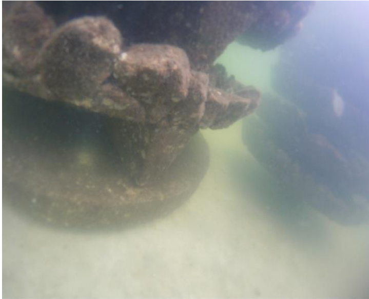
Figure 18-Two types of Ecodisc design- "Table Tops" (left) show a concrete pad stabilizing the units and the "Lillypads" with the piling exposed and secured by a collar underneath.
