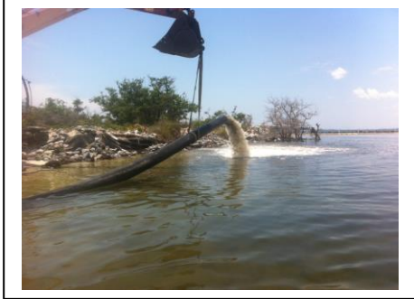
Figure 26: Sand being piped from the spoil site to Deadman's Island
