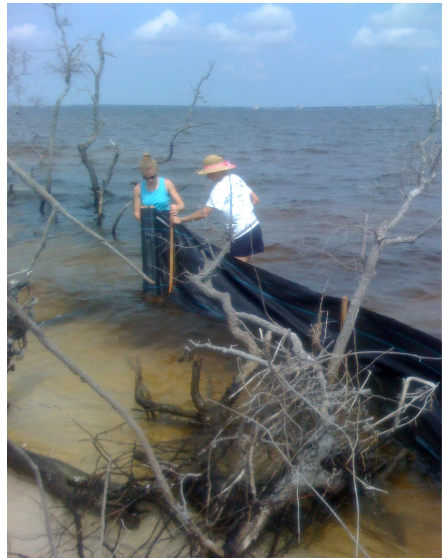
Fig. 17 – Volunteers placing temporary shoreline protection 2008
