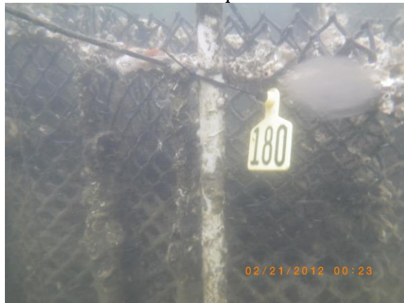
Figure 16: 2012 -Reefs completely barren and all oysters are no longer attached to the mesh bags. which creates an ineffective breakwater.
