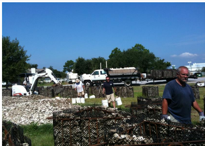
Fig.19 – mass amount of fossilized and recycled shell for the breakwaters
