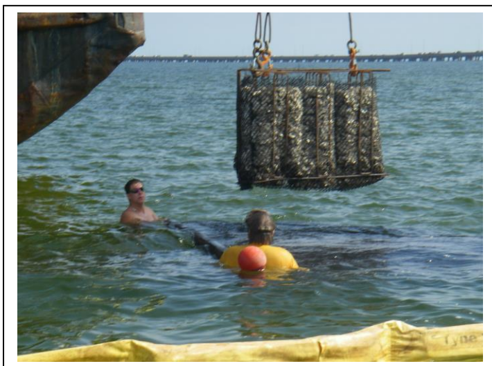
Figure 13: These rebar breakwaters designed by Coastal Environments were required by the regulatory agencies, to be placed below mean high water as opposed to above mean high water as the later breakwater design
