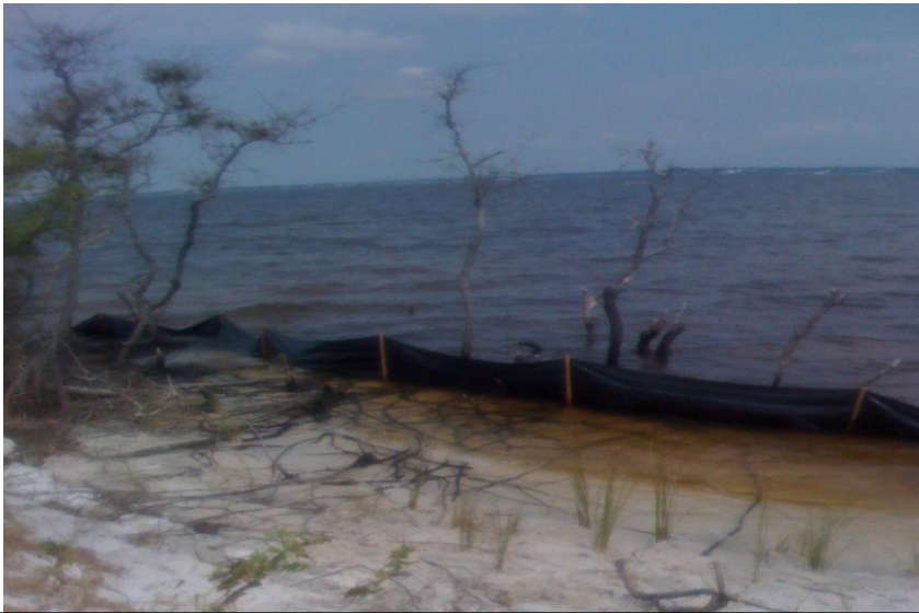
Fig. 16- a bandaid attempt of shoreline protection to allow plants to become stabilized 2008
