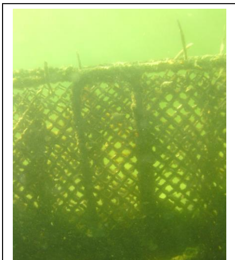
Figure 17: November 2013 The loss of shell inside the mesh bags of the rebar breakwater units.
