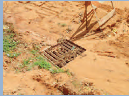
Drain gate allows direct sediment pollution to the river and bay along Rattlesnake Bluff Road. © TNC
