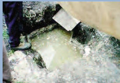
Cesspits (pictured) and septic tanks leach nutrients and pathogens into Keys' nearshore waters. © TNC
