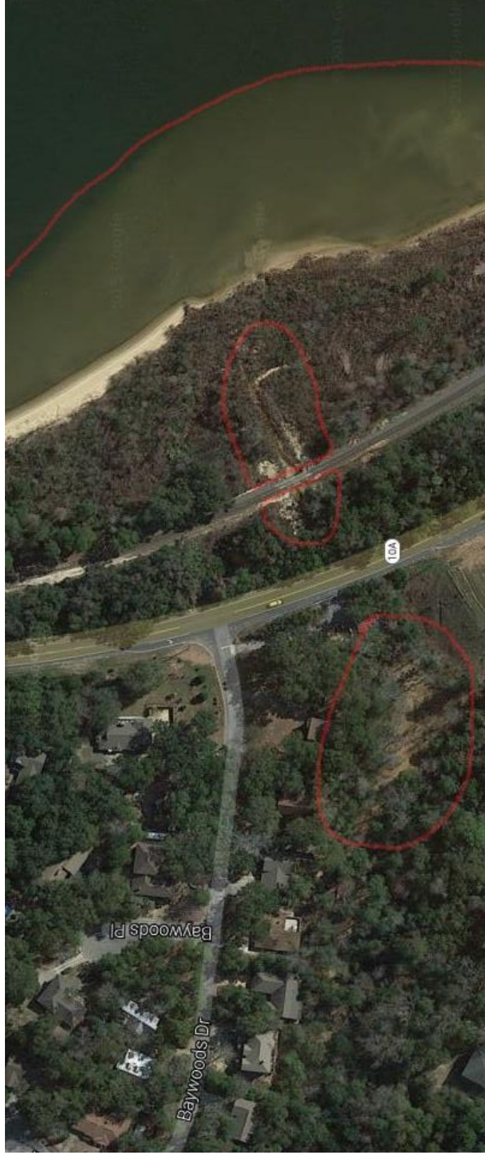
Post-storm even aerial. Sediment deposits downstream are starting to impact vegetation. Increased sediment upstream and downstream of Scenic Highway and CSX Railroad into Pensacola Bay.
