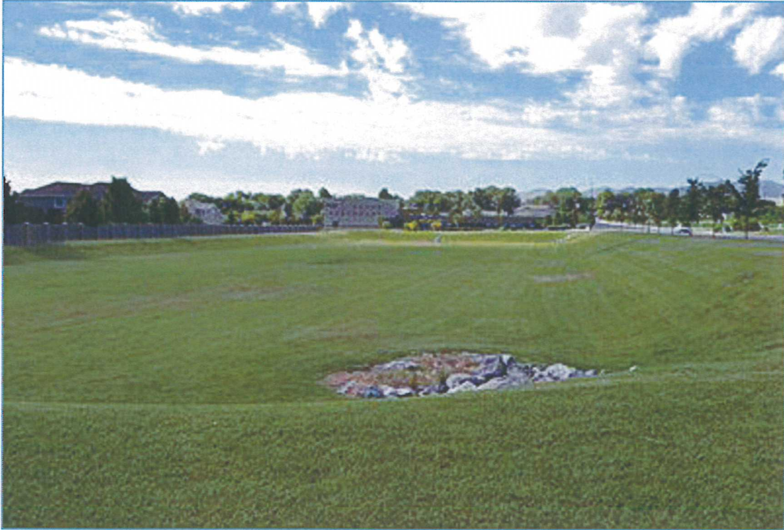
District Detention Basin Park, South Jordan, Utah
