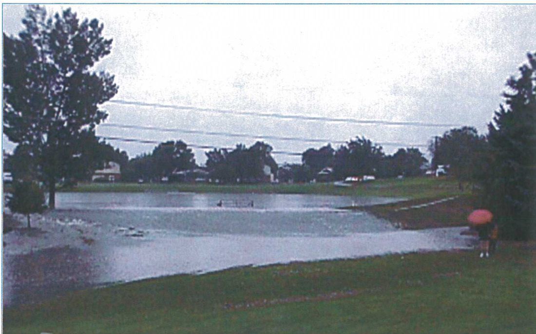
Powers Park Detention Basin Park, Littleton, Colorado, during 8/17/2000 rain event. Photo taken by Littleton City Engineer Bob Deeds.
