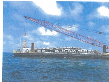
Re-use concrete poles/bridge materials
