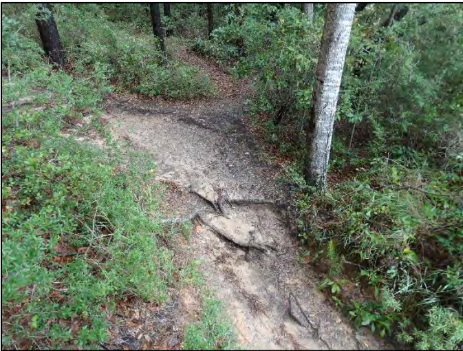
Above: Erosion to the left of the north side of the boardwalk.
