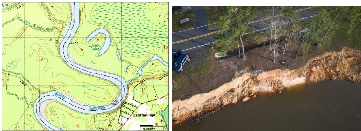
Figure 1. a) Topographic map of the Estiffanugla area in the 1980s shows several houses both west and east of the road adjacent to the river; b) Drone photograph of the eroding bluff at Estiffanugla taken March 2016 is a short distance from a road and houses. Signs of active erosion include fallen fence post and tension cracks, eroded sediment blocks, an overhanging fence line and a few eroded trees at the base (Photograph taken by Scott Walls).
