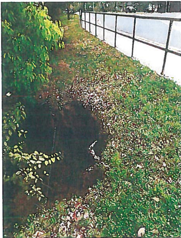
Collapsing areas encroaching toward roadway
