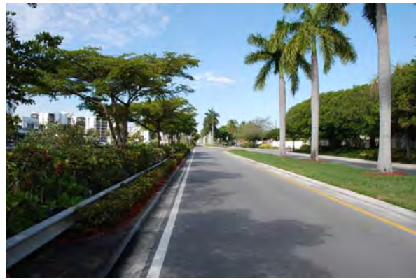
NE 207 th Street Looking West
