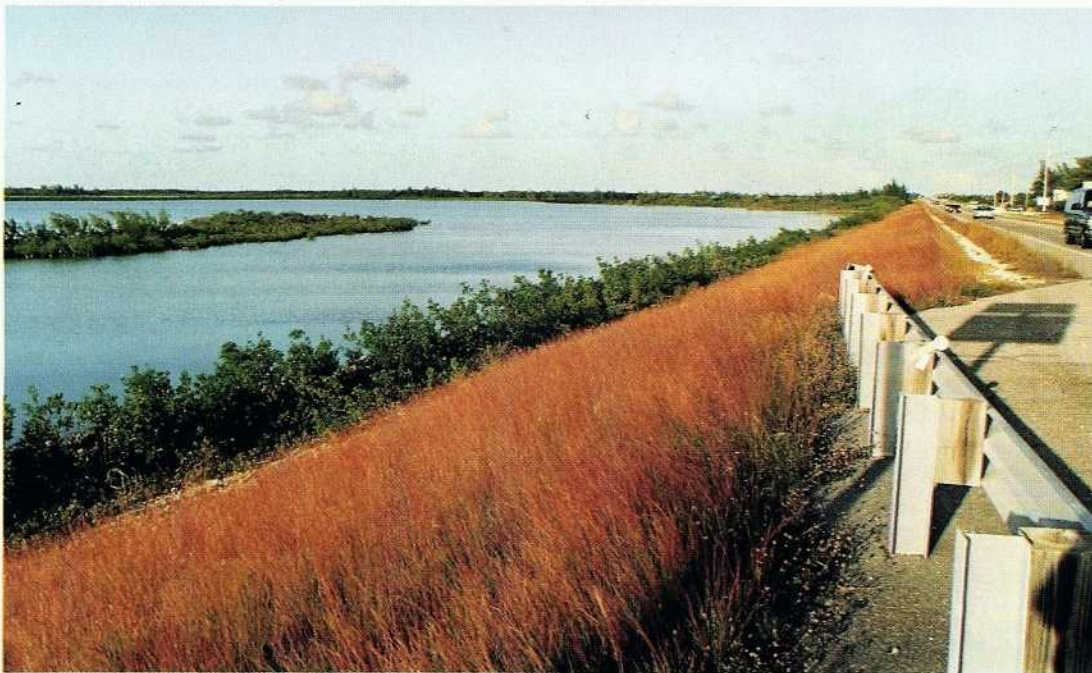
Figure 15. Lower Sugarloaf Channel, grassed slope, Miami Gulf side, view east, 11/92.
