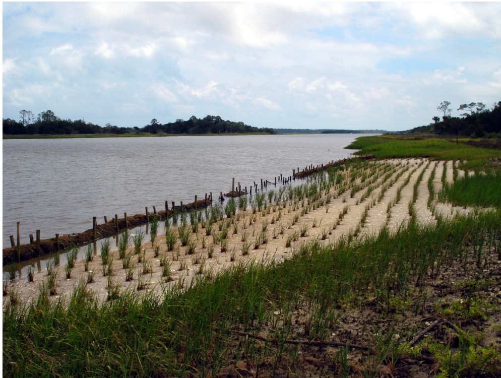
Photograph C6.2 Marsh Restoration in St. Johns County, FL
