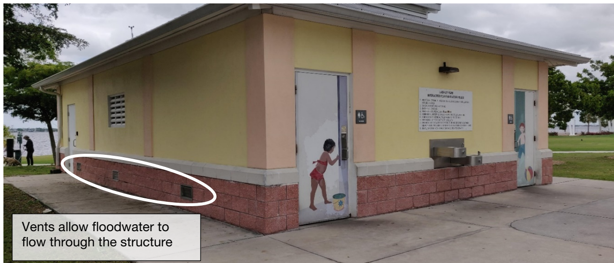
Photograph 4.1 Wet Floodproofing (Accommodate Strategy) at Laishley Park
