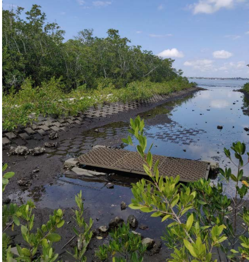
Photograph 4.6 Drainage Culvert along Punta Gorda's HarborWalk
