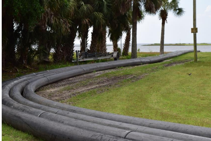
Photo 3 - Dredging equipment stationed outside coastline
