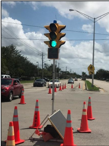
Temporary solar traffic signals in Coral Springs after Hurricane Irma. (Image courtesy of Coral Springs Police.)
