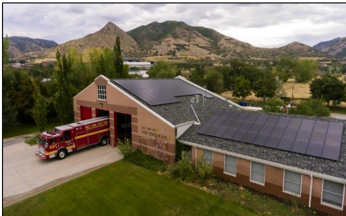
Salt Lake City Fire Department with Solar Panels.
