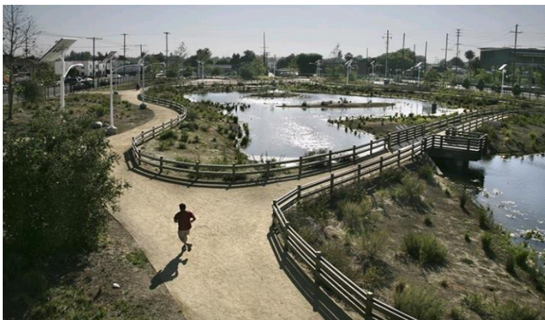
Stormwater Park as Community Amenity (Image courtesy of Architecture Magazine.)
