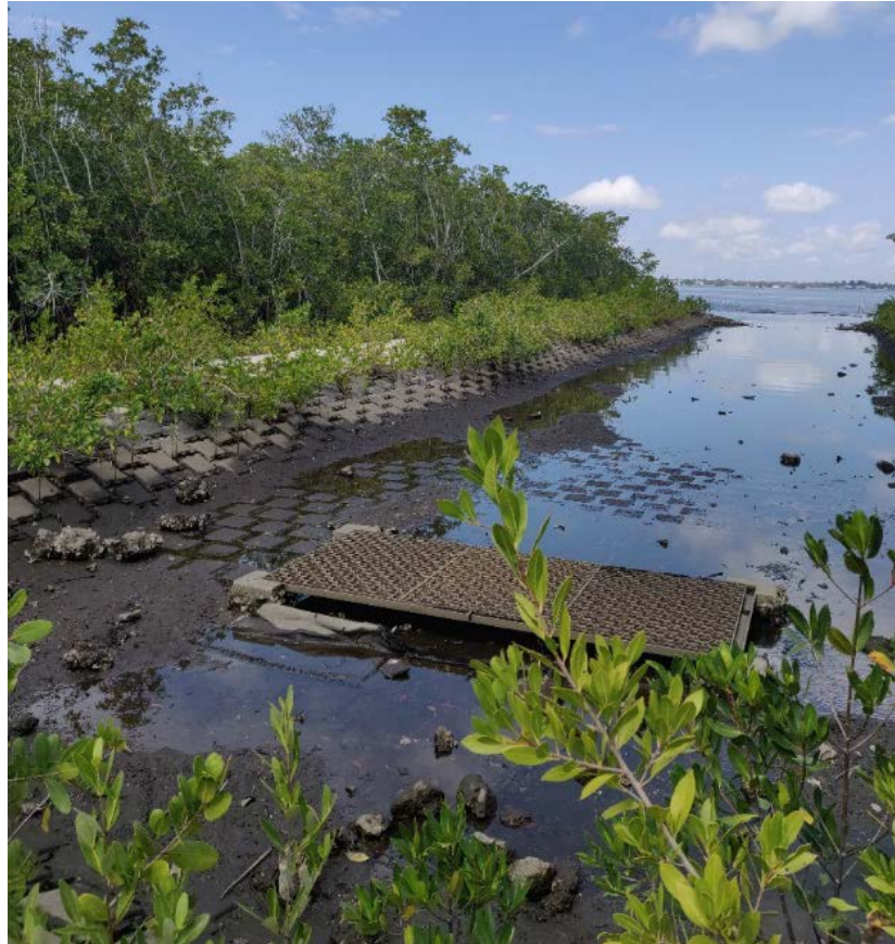
Photograph 4.6 Drainage Culvert along Punta Gorda's HarborWalk
