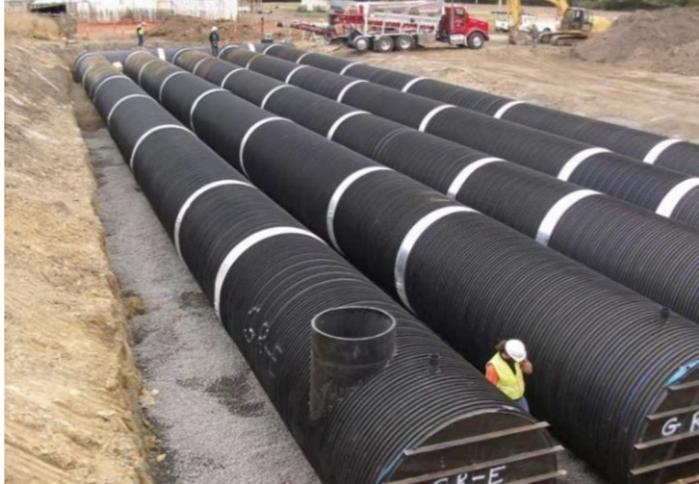
Photograph 4.5 Storage Tanks for Excess Runoff ( www.conteches.com )
