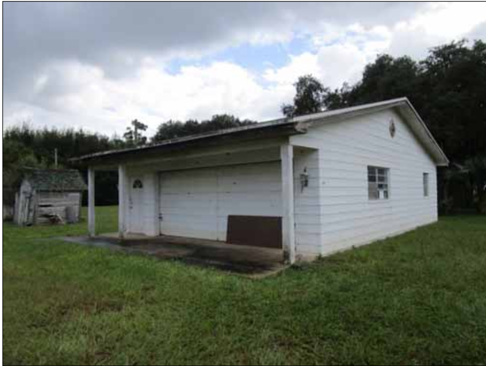
VIEW LOOKING SOUTHEAST AT THE DETACHED GARAGE
