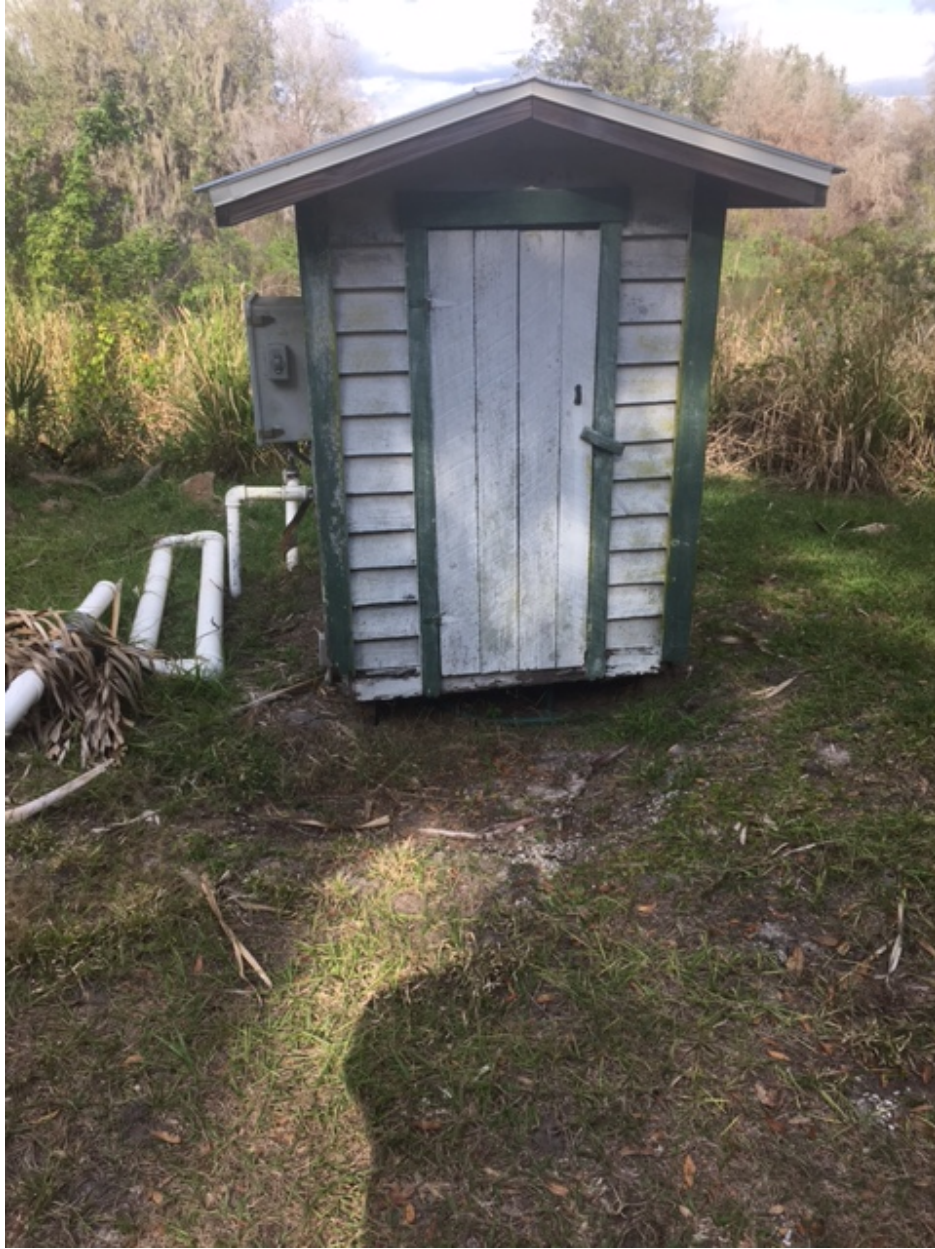
View to the North of Pump House located adjacent to the Northern periphery of Tract No. 19 103-837.
