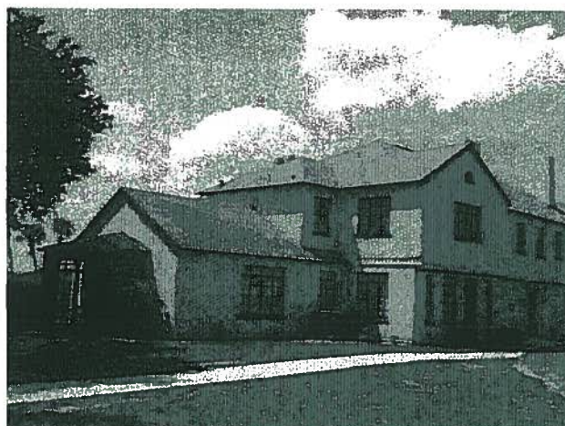
Northeast Elevation (Detail)
