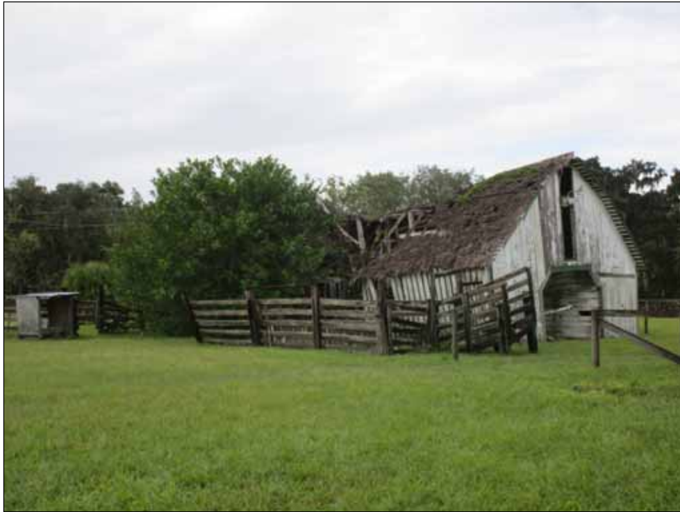
VIEW LOOKING NORTHWEST AT THE BARN
