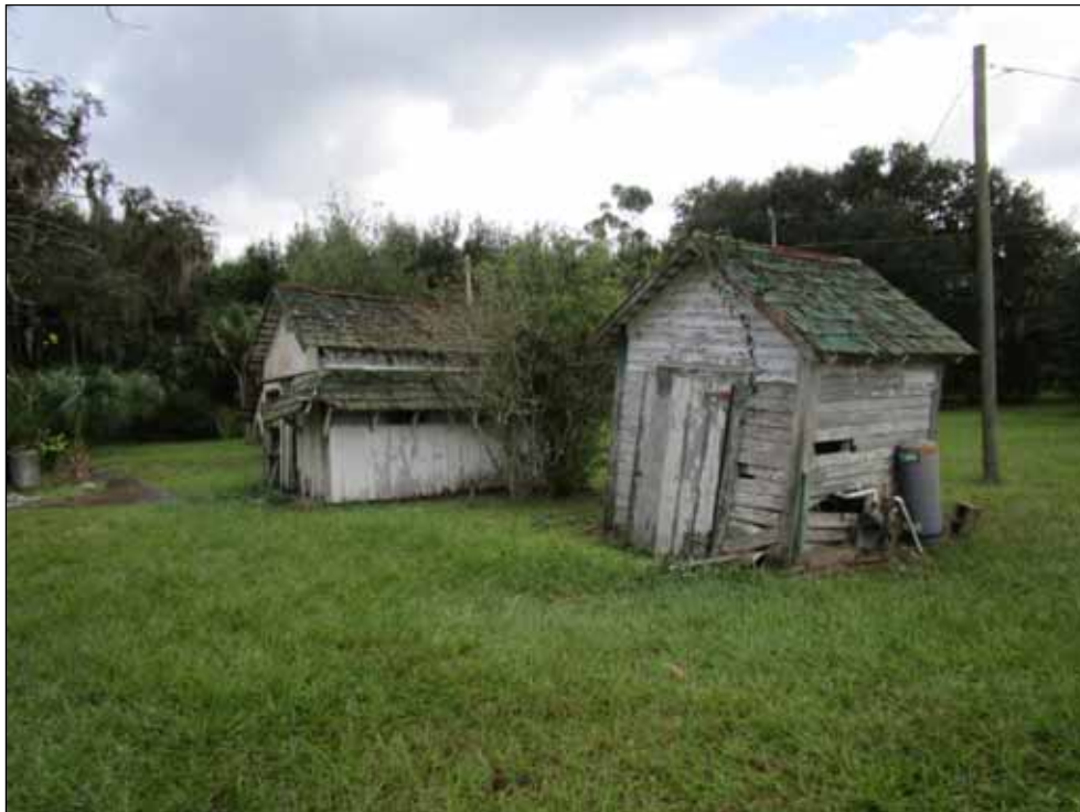
VIEW OF PUMPHOUSE AND SHED
