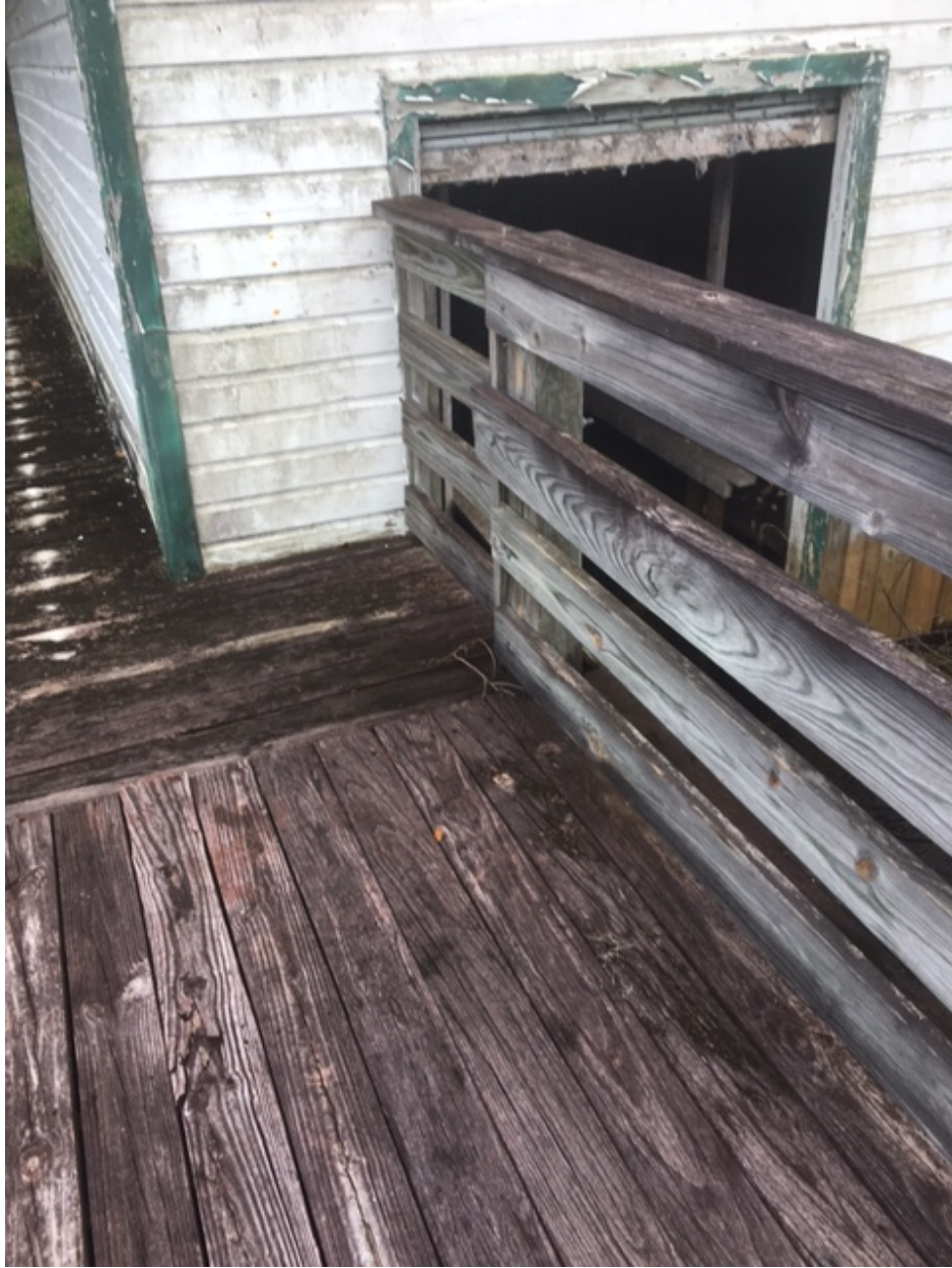
View of Boat House and Boat Dock located adjacent to Northern periphery of Tract No. 19 103-837.
