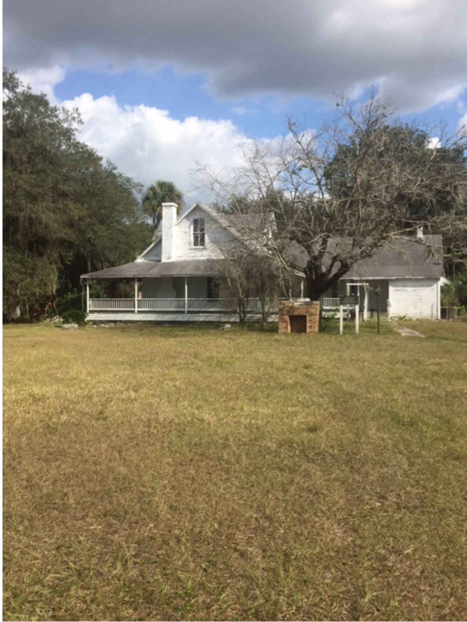
View to the North of Main House located within Tract No. 19 103-654.
