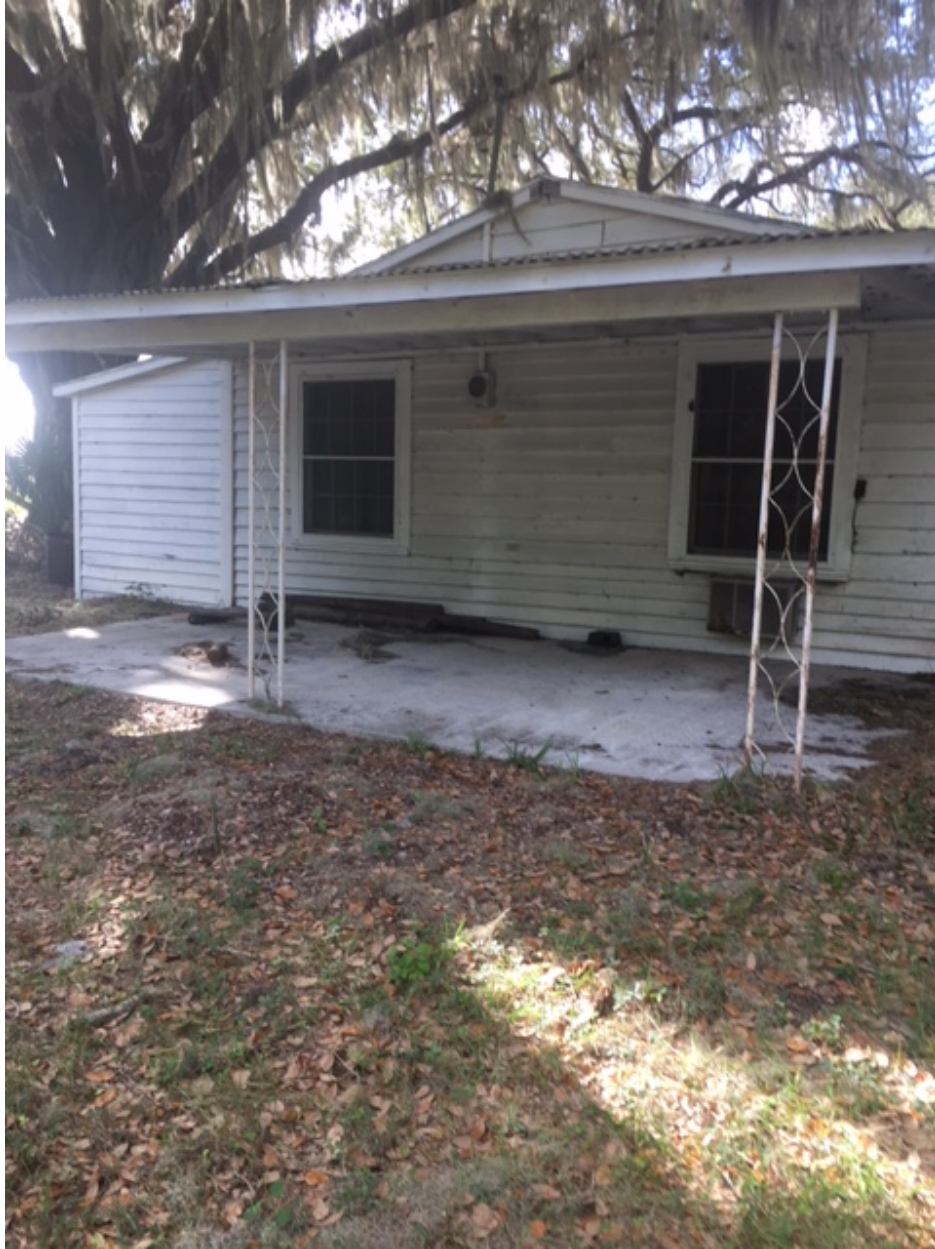
View to the South of the Guest House/Caretaker's Residence located within Tract No. 19 103-654.
