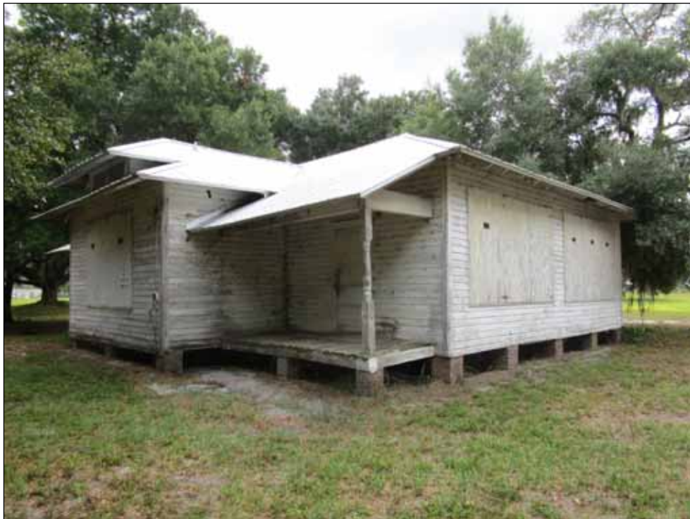
VIEW LOOKING SOUTHWEST AT THE SCHOOL HOUSE
