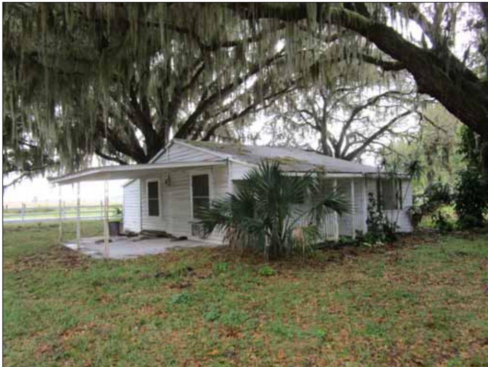
VIEW LOOKING SOUTHWEST AT THE GUEST HOUSE
