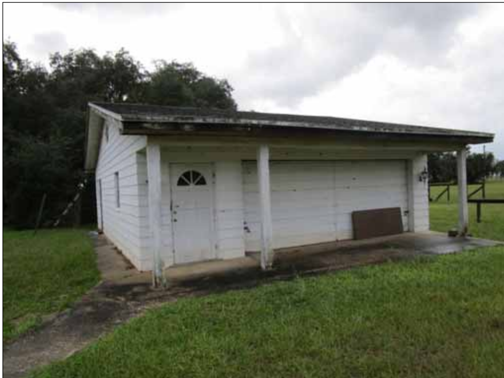
VIEW LOOKING SOUTHWEST AT THE DETACHED GARAGE
