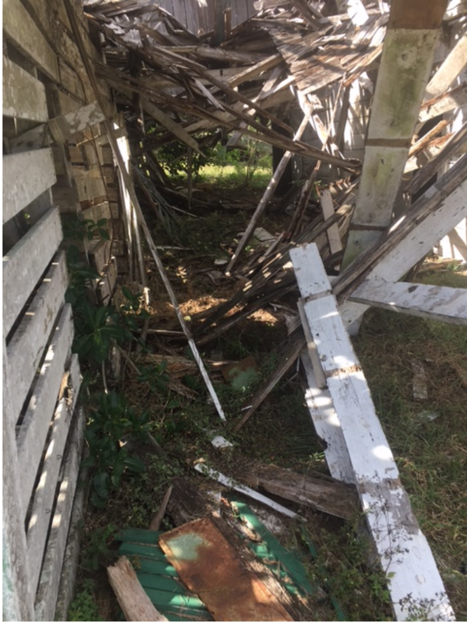
Partial view to the South of the interior of the Barn.
