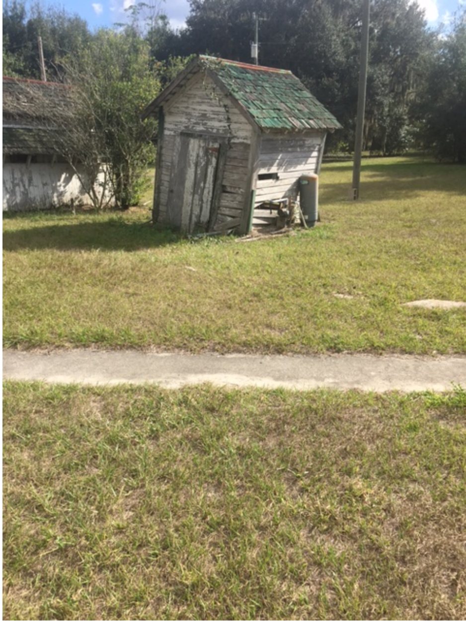
Additional view of Pump House and Storage Shed.
