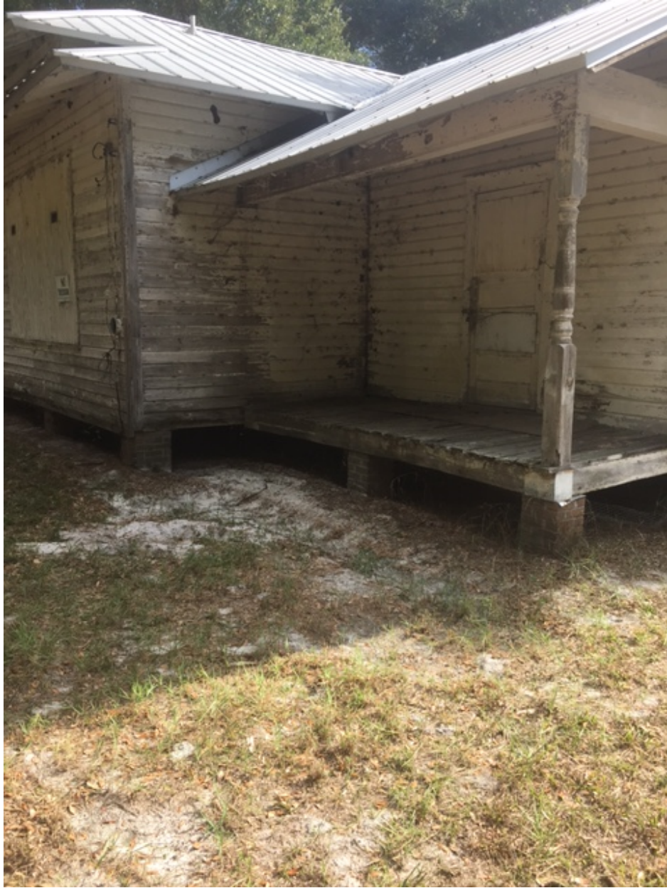
Additional view of exterior of School House.
