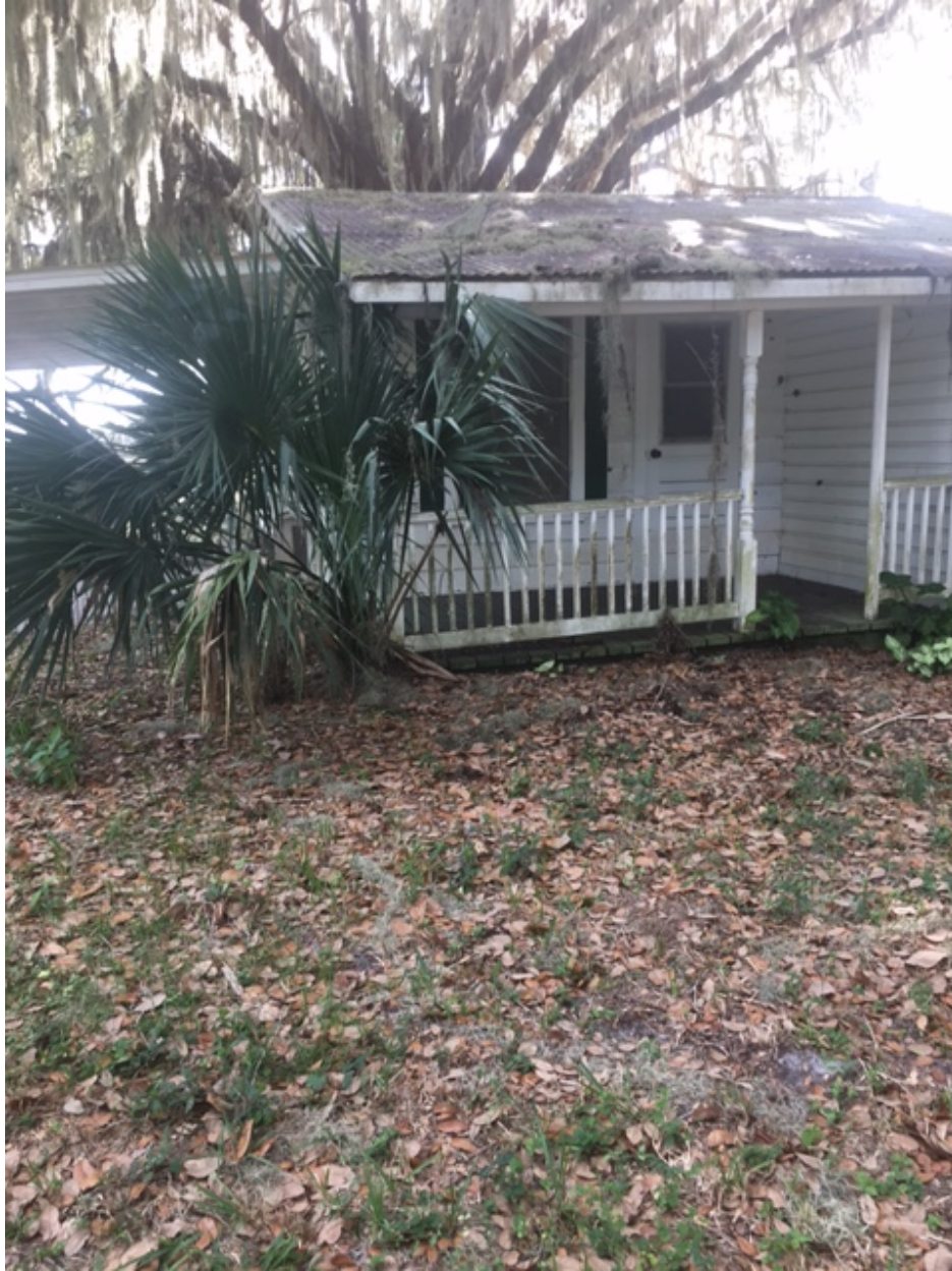
View to the East of the Guest House/Caretaker's Residence. Note the settling of the structure.
