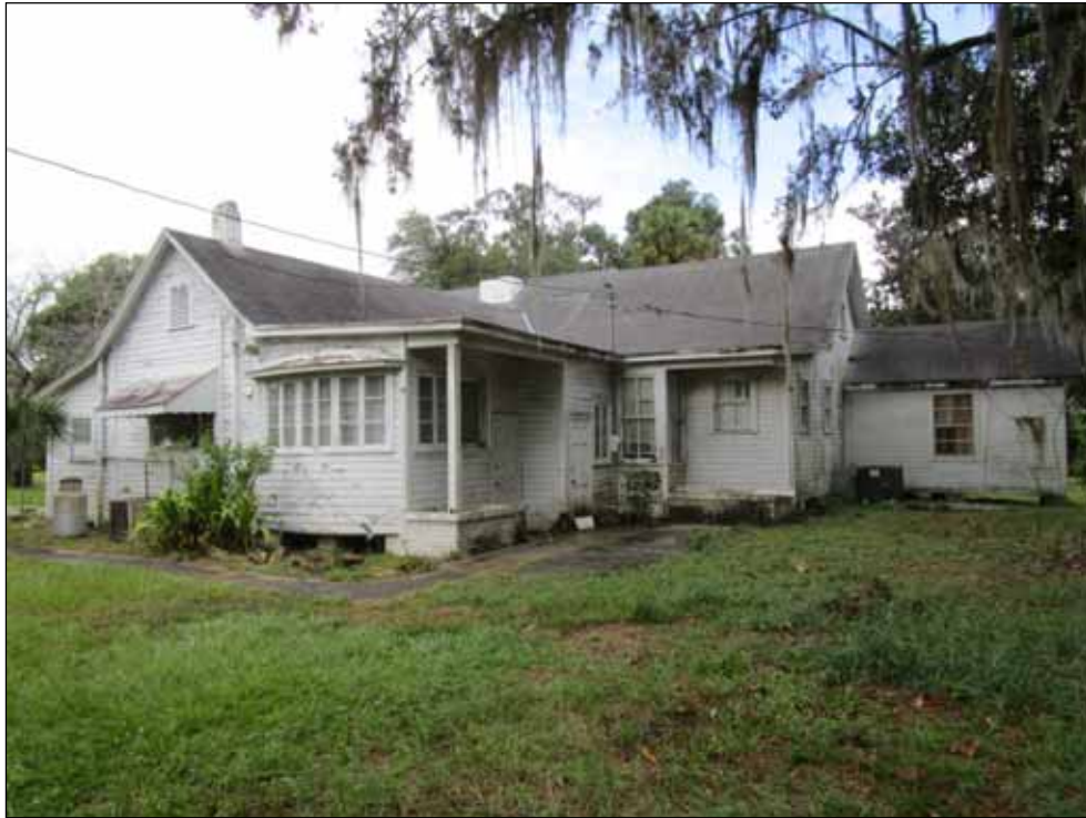
VIEW LOOKING NORTHWEST AT THE SINGLE FAMILY RESIDENCE
