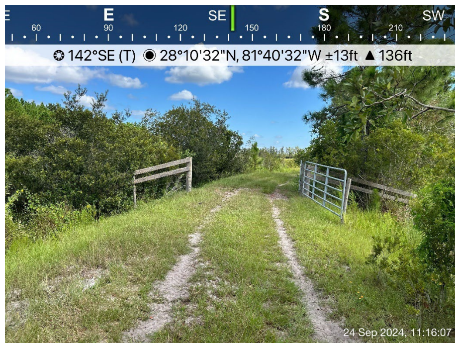
Photo 40: Typical access road and gate on the Subject Property.
