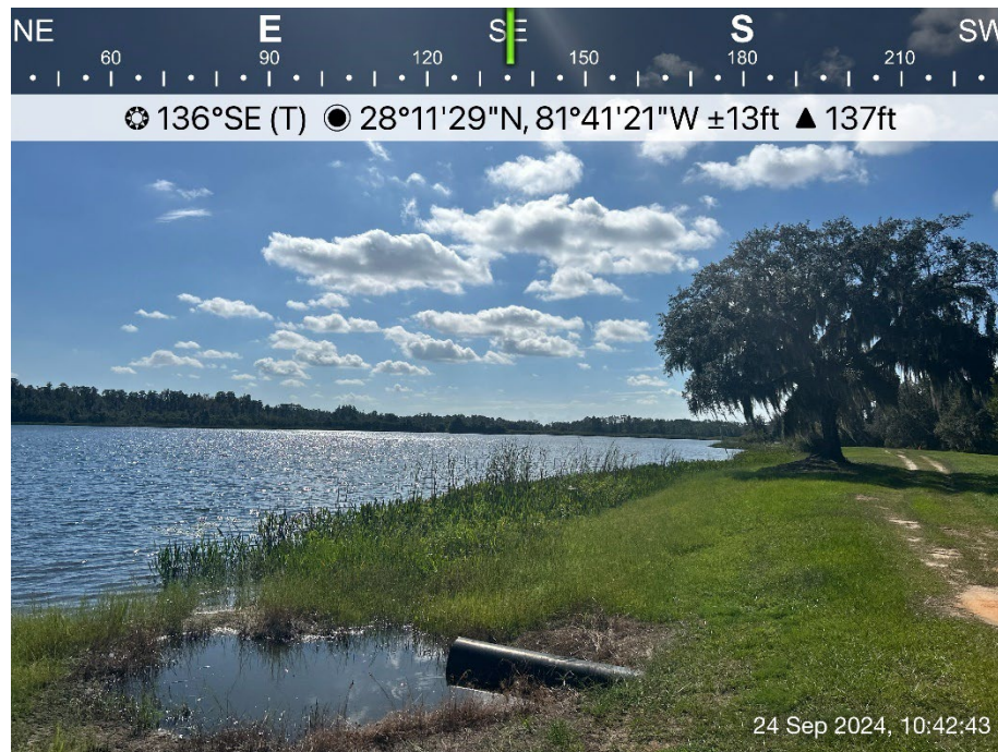
Photo 35: Culvert under access road observed on the Subject Property.
