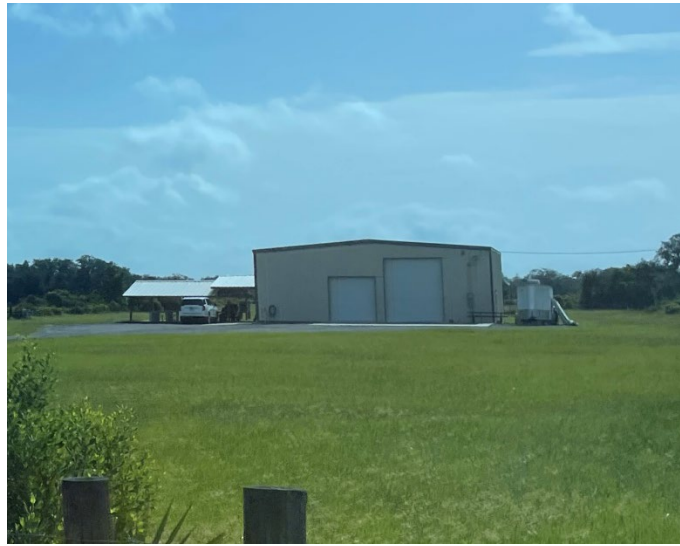
Figure 6. Large, Central, Air-Conditioned Facility with Patio
