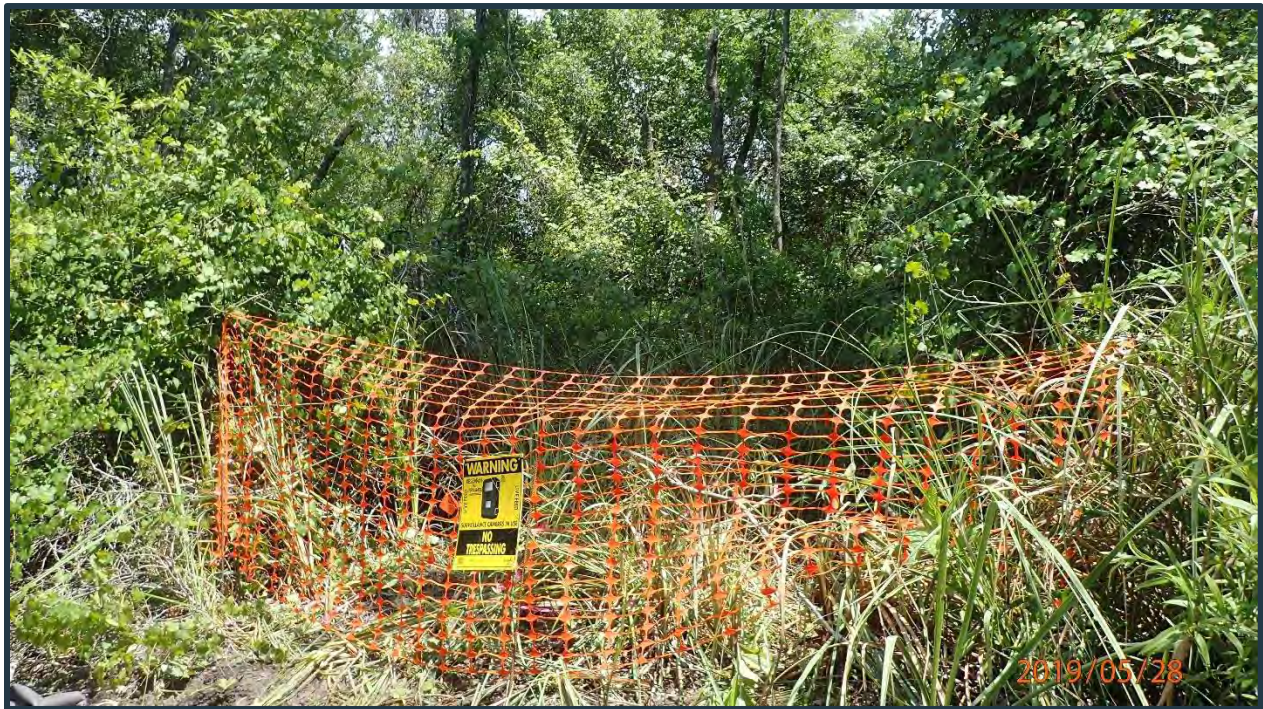
Figure 4.4 – Construction Fence Barrier
