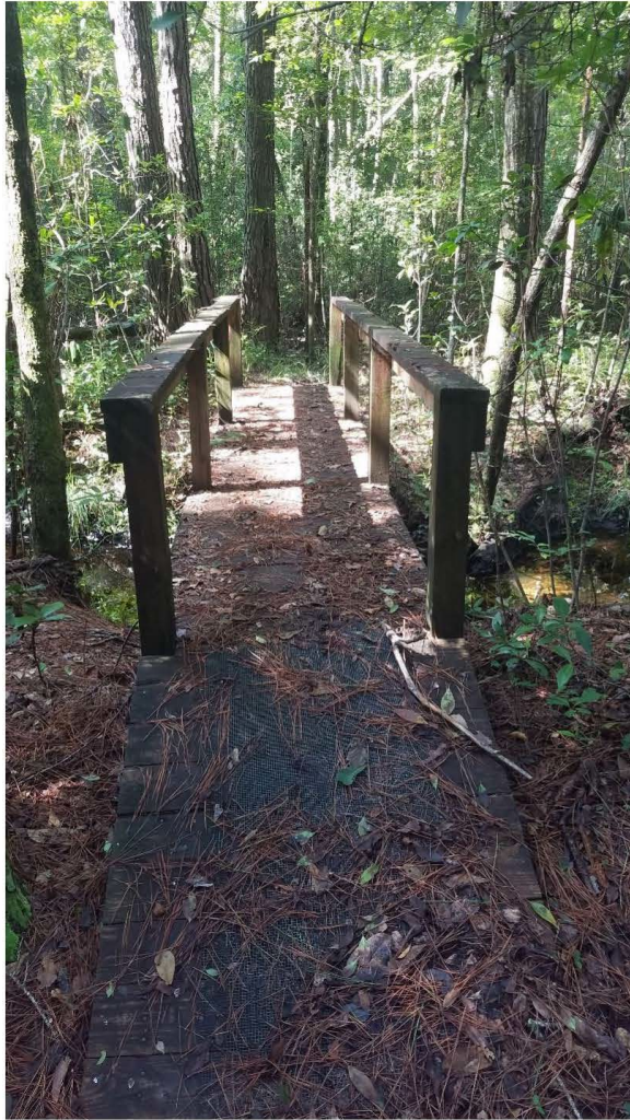
Current west bridge, photo taken south facing.
