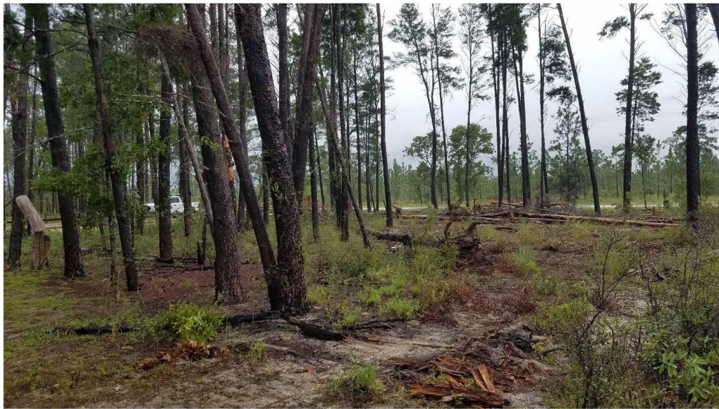
North facing photo of parking lot expansion, Lines Tract, Lake Talquin State Forest.
