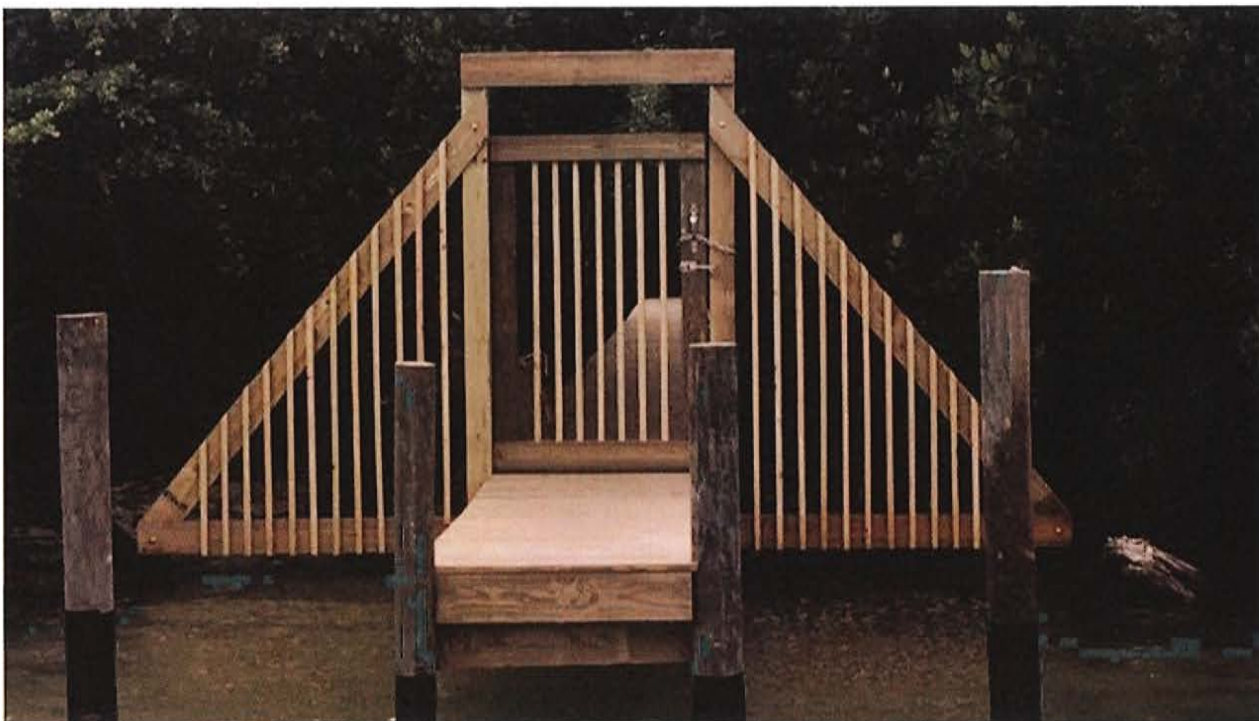
Rebuilt bayside dock and boardwalk in the "Narrows" section of Cayo Costa Island. Photo Special To The News-Press
