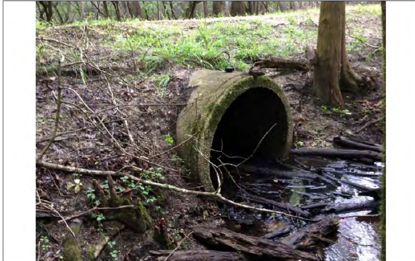
Photo No. 4b. Culvert location; view of the easternmost culvert (August site visit). View to the northeast.
