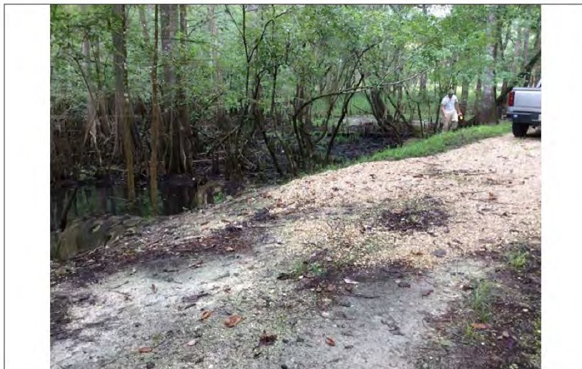
Photo No. 5a. View of culverts from low point in access road (August site visit). View to the southwest.
