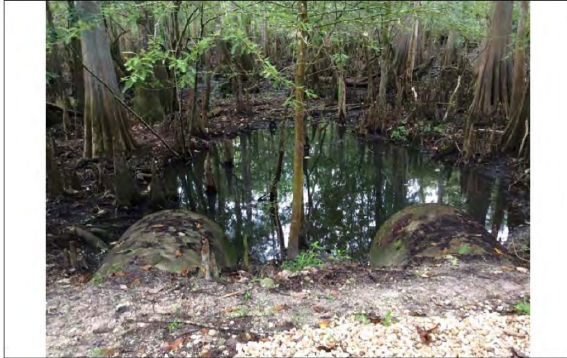
Photo No. 5b. Culvert location (August site visit). View to the north.
