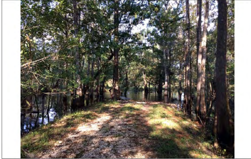
Photo No. 12a. Culvert location; view towards low point in access road (September site visit). View to the west.
