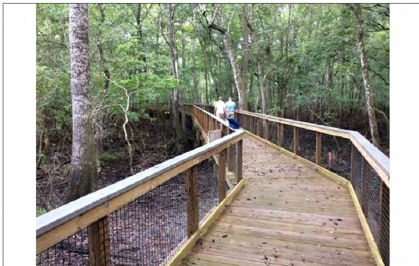
Photo No. 2. Boardwalk location (August site visit). View to the west.
