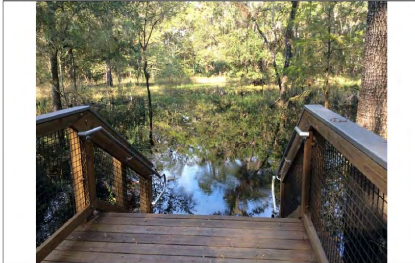
Photo No. 15. End of boardwalk (September site visit). View to the west.
