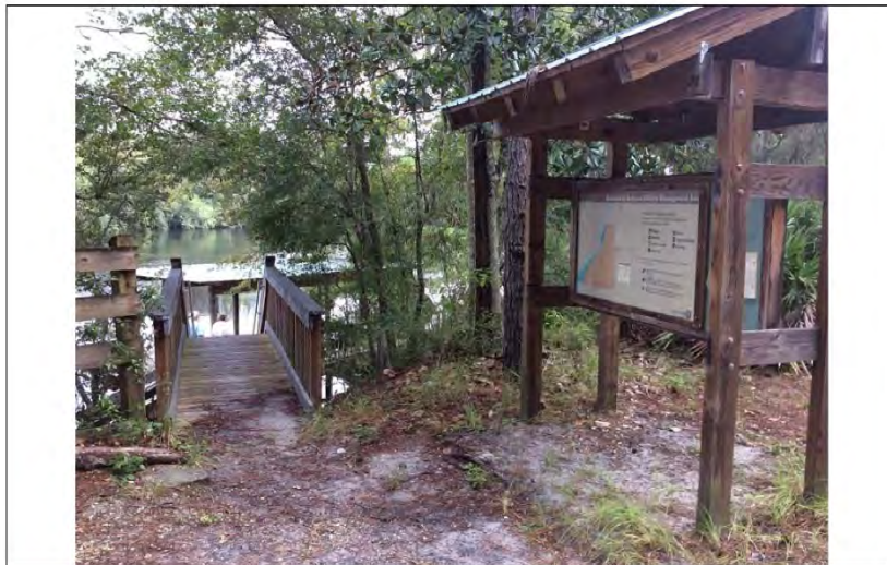
Photo No. 8. Dock location (August site visit). View to the north.
