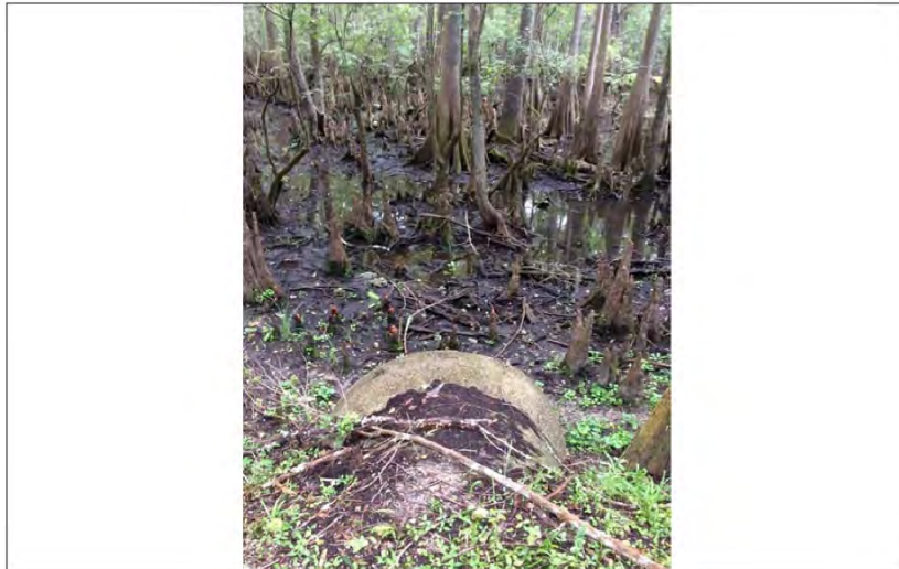
Photo No. 6. Culvert location; view of westernmost culvert (August site visit). View to the south.
