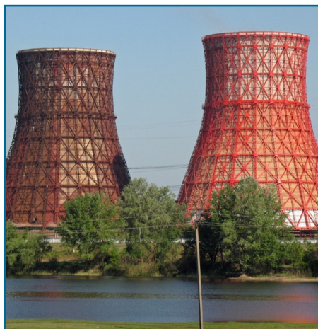
Figure 5. Hyperbolic Cooling Towers (Source: Victor Vizu).
