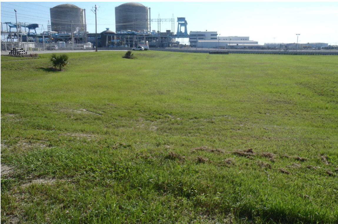
Figure 4. Existing conditions at St. Lucie Substation, facing east.
