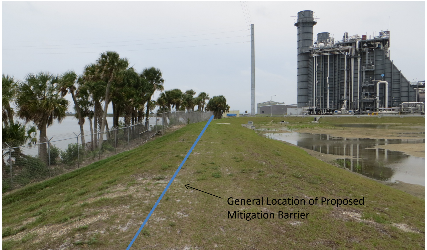
Photo 1 - East Embankment of Pond C (Looking South)
