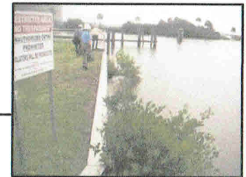
PHOTO 2: EXISTING CONDITIONS AT LOCATION WHERE PIPING CROSSES SEAWALL
