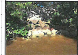
PHOTO 1: EXISTING CONDITIONS AT LOCATION WHERE DETERRENT WALL ABUTS SHORELINE
