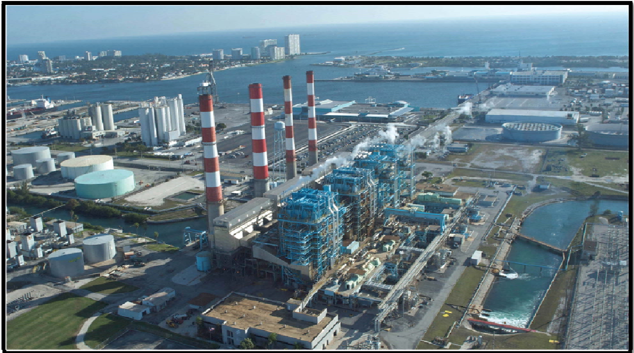
Existing Port Everglades Plant
