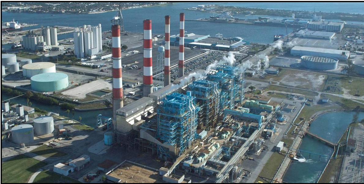
Figure 3. View of Existing Port Everglades Plant Units 1-4 (Provided by FPL)
