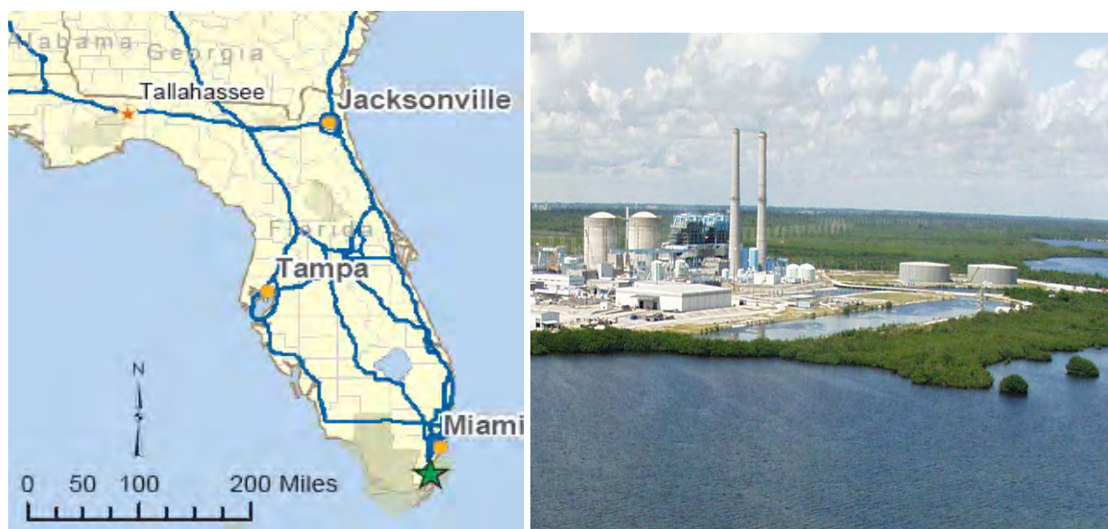
Figure 1. TPP General Property Location and Site Photo. (Florida Power & Light)
