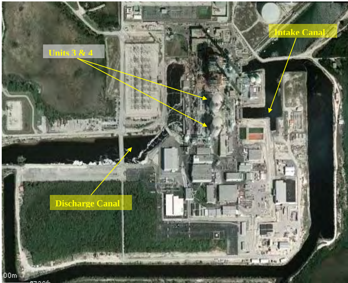
Figure 6. Aerial View of Turkey Point Plant Showing Intake and Discharge Structures. (2008 Yahoo! Inc., identifiers added by SCO)
