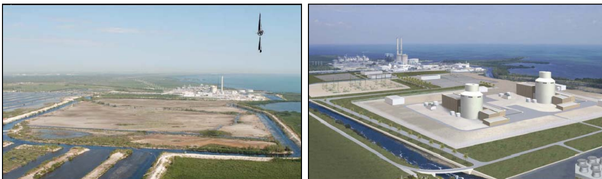
Figure 3. Aerial of Units 6 & 7 Site and Conceptual Illustration (Looking Northeast) Depicting the Completed Units and Immediate Supporting Structures (FPL SCA Figs. 4.2-1 & 4.2-3)
